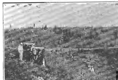
Typical cut-over lands on the Olympic Peninsula, Washington, where land clearing is being done with a tractor equipped with a bulldozer. The stumps are mechanically shoved out.
