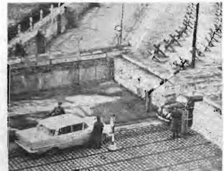
A carcheck at one of the gates in "The Wall."
