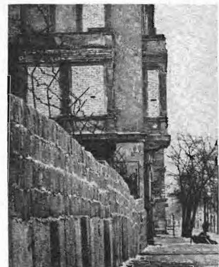
Walled-up windows on the boundary line of "The Wall."
