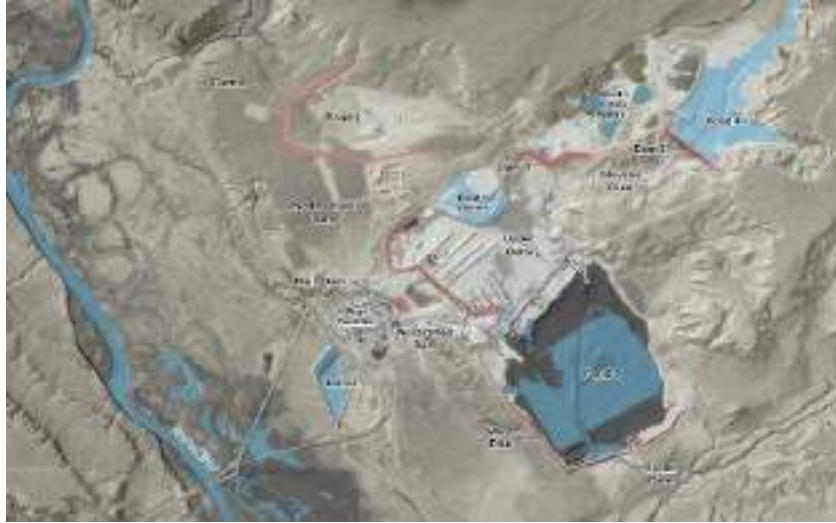
Source: Barr-Ciner-2020_Dam-Safety-Report_20210224-signed.pdf Figure 17.1 Sisecam Tailings Impoundments and Evaporative Ponds
