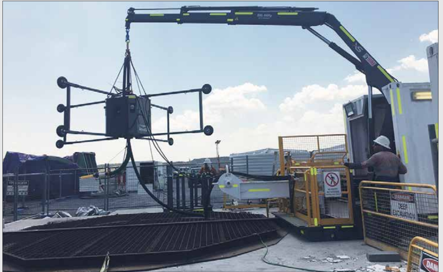
Mancala provides unique solutions for shaft construction and ancillary services.
