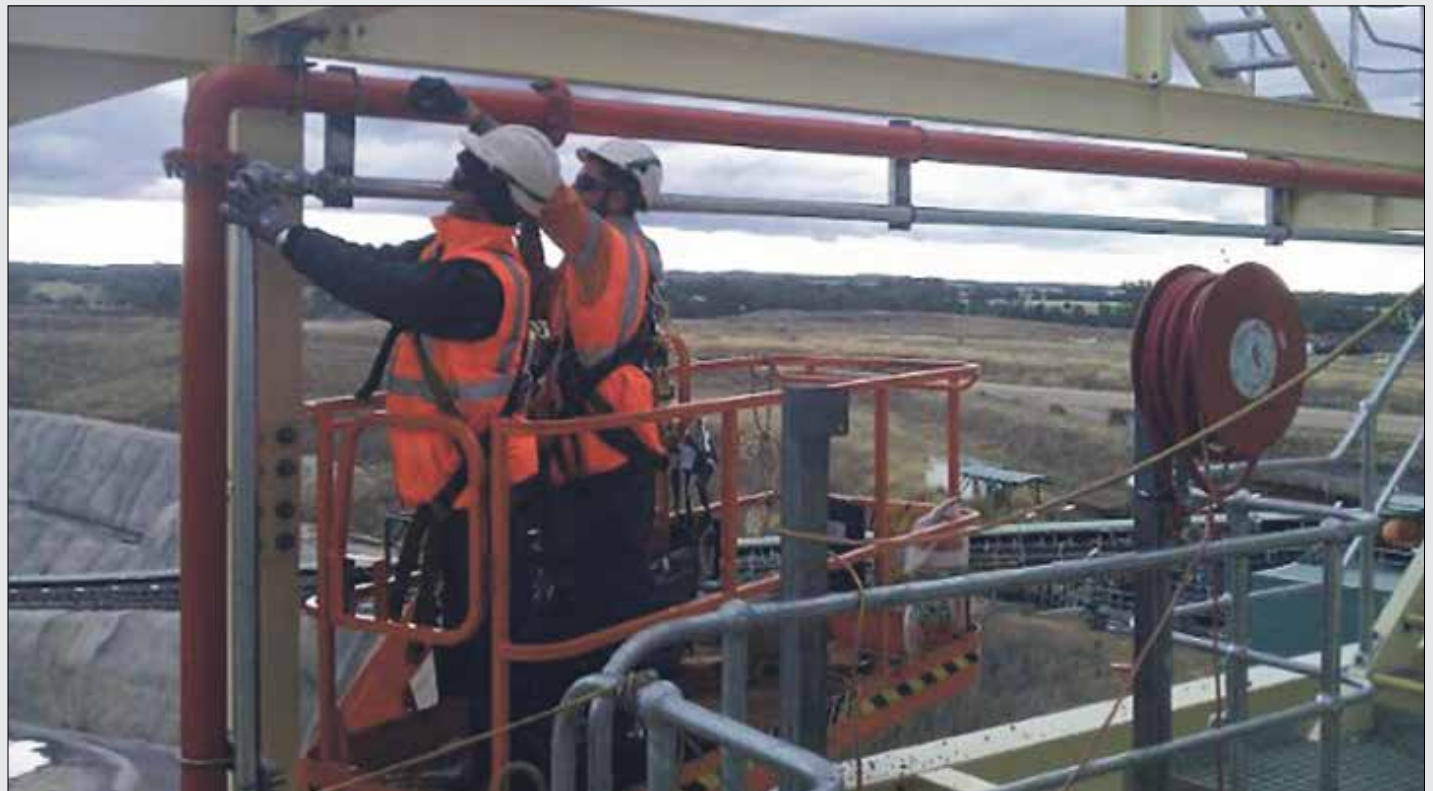
The company has the capacity to undertake highly specialised projects.
