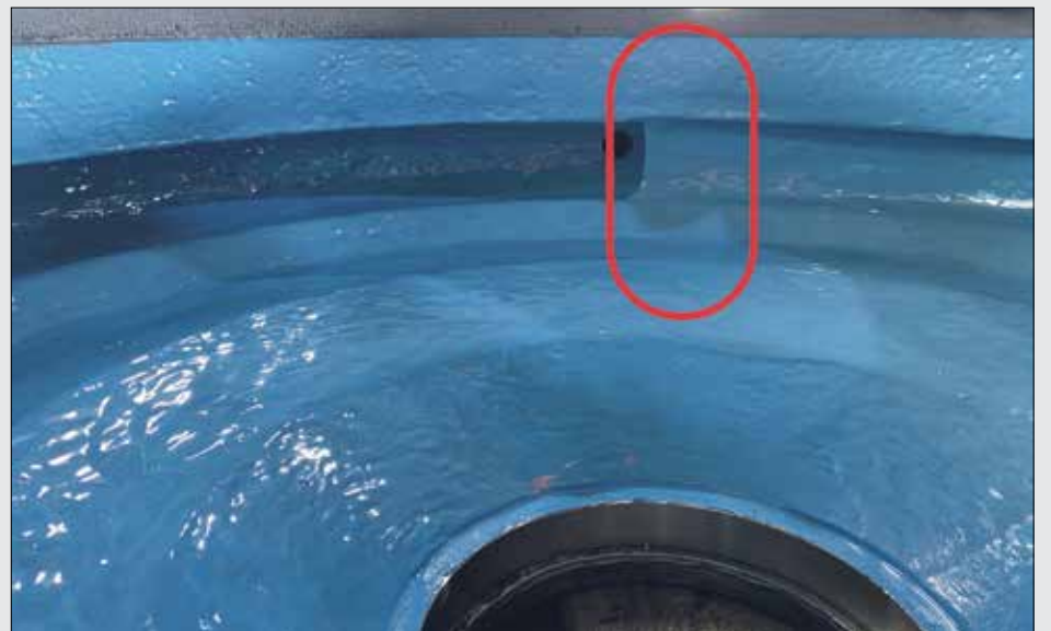
The same cut water after repair.
