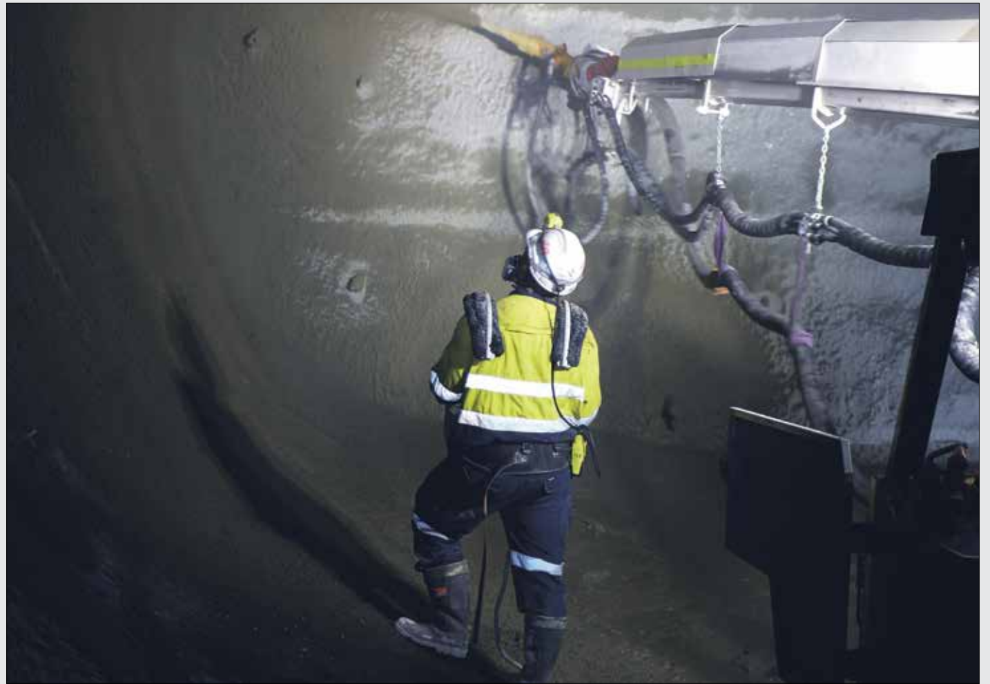
Redpath uses advanced shotcrete methods in all its operations.
