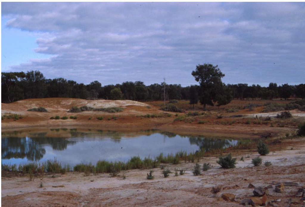
Plate 2.3: Quinn's Dam, Gluepot Reserve. The dams or in-ground tanks in the study area are characteristically placed in natural depressions which may collect water after rain, and have four walls constructed from soil excavated from within the dam. Water enters the dam through one or more drainage channels which are dug into the surrounding area (pictured on far side of dam). Note the surrounding Casuarina pauper .
