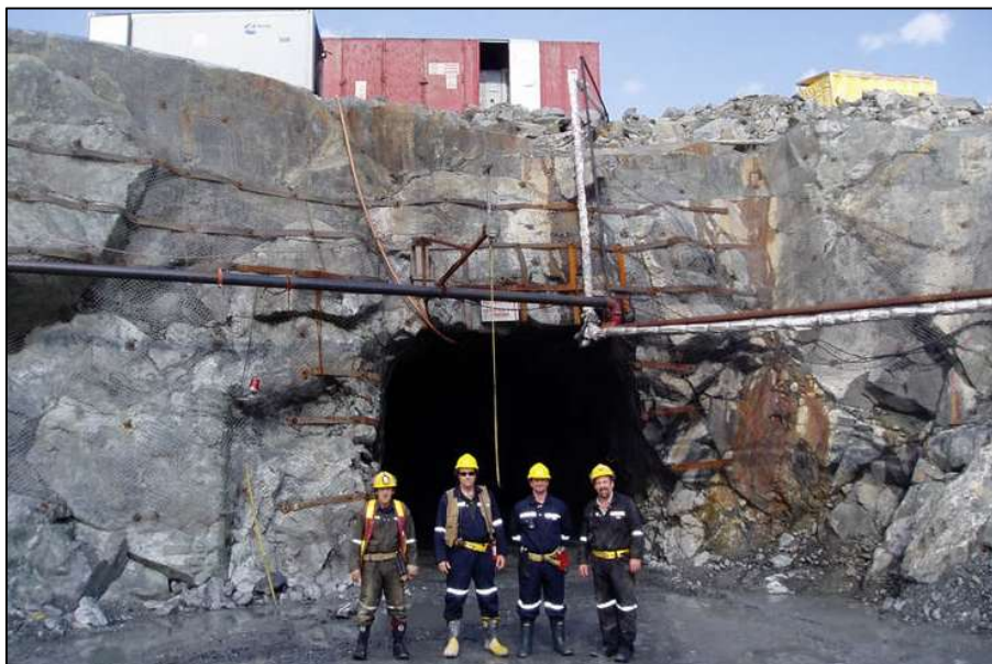
Figure 6.8 – Portal of the ramp started in the north wall of the open pit (from Balmoral's website)
