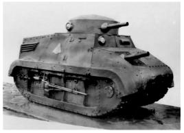
Carro de Combate de Infantería 1937 (Tier II Light Tank) Minimal armor, vulnerable to small arms fire on its flat side. Good parameters in everything else, armed with a 20mm Breda. Pretty agile and speedy. One vehicle, suspension taken from an Italian prototype.
