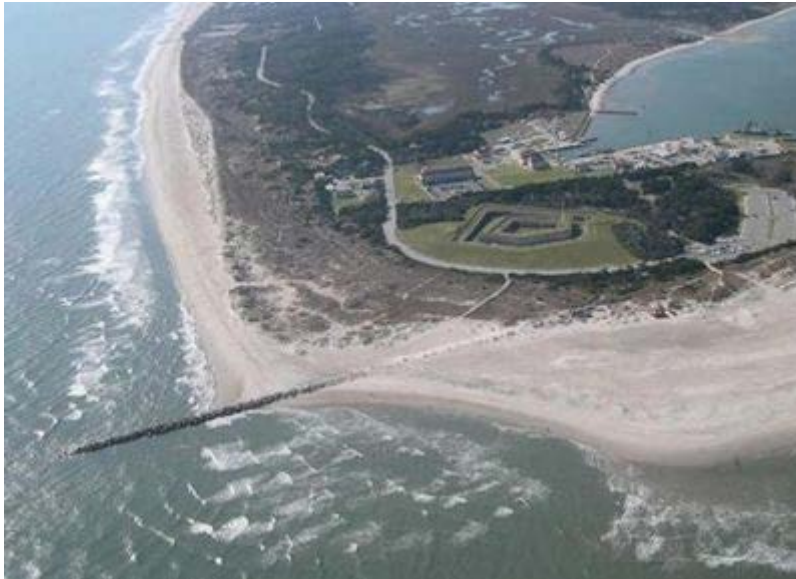
Figure 32. Terminal groin at Fort Macon State Park beach in North Carolina.
