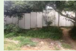
Existing Pond inside site → hard barricaded to protect from construction activities
