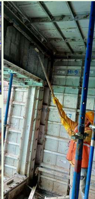
The person using the curing compound
