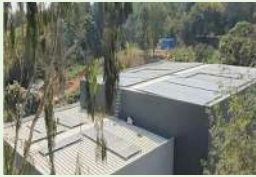
Positioning and constructing new site establishments carefully between existing trees to protect them
