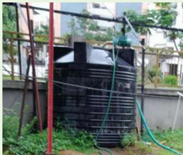
Rainwater storage and reuse for curing
