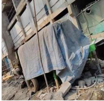
Use of electric concrete pumps (Mahindra Alcove, Mumbai)
