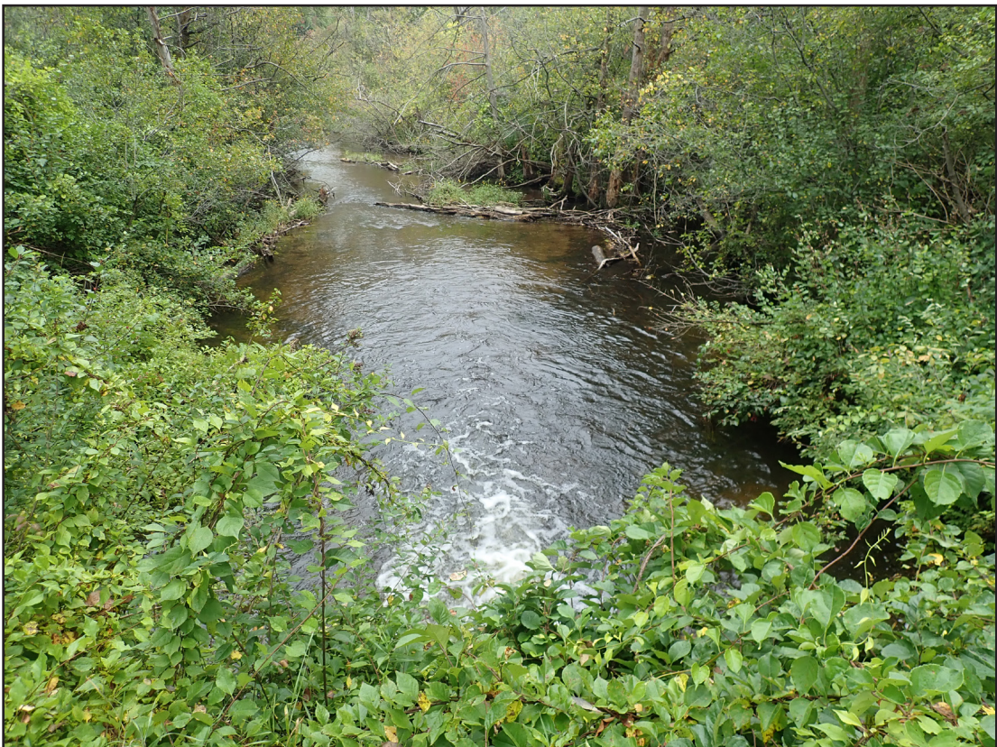
Photo 12. Looking downstream from the culvert and stream crossing.
