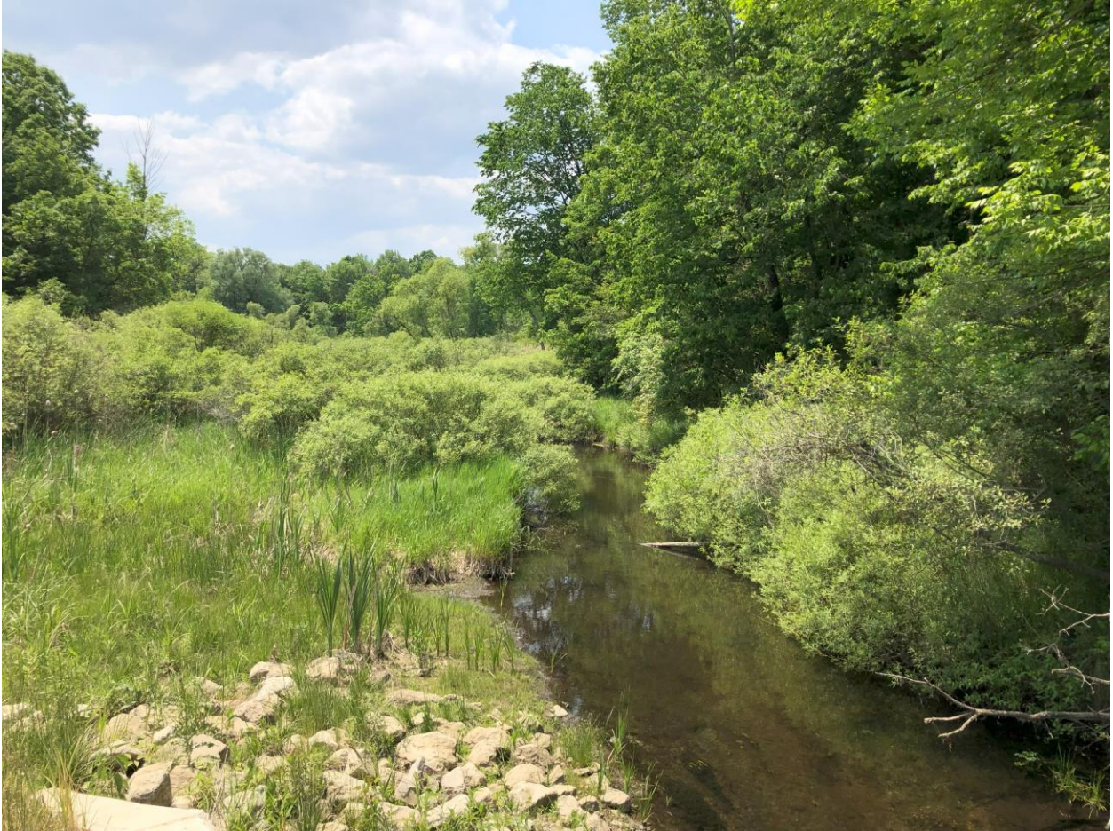
Figure 13. The South Branch Flint River stream crossing consisted of a bridge with large rock riprap lining the embankment – looking west. Turtles typically inhabit permanent waters such as lakes, ponds, or slow-moving rivers. Photo by Michael A. Sanders.
