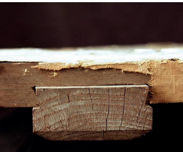
Fig. 6. Side view of the wooden panel showing the crosspiece strengthener
