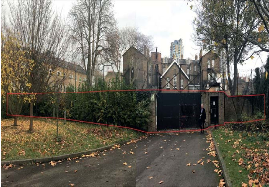
Figure 1: The 34 metre stretch of the boundary wall to IWML, as seen from within Geraldine Mary Harmsworth Park, which forms the north western perimeter to the application site
