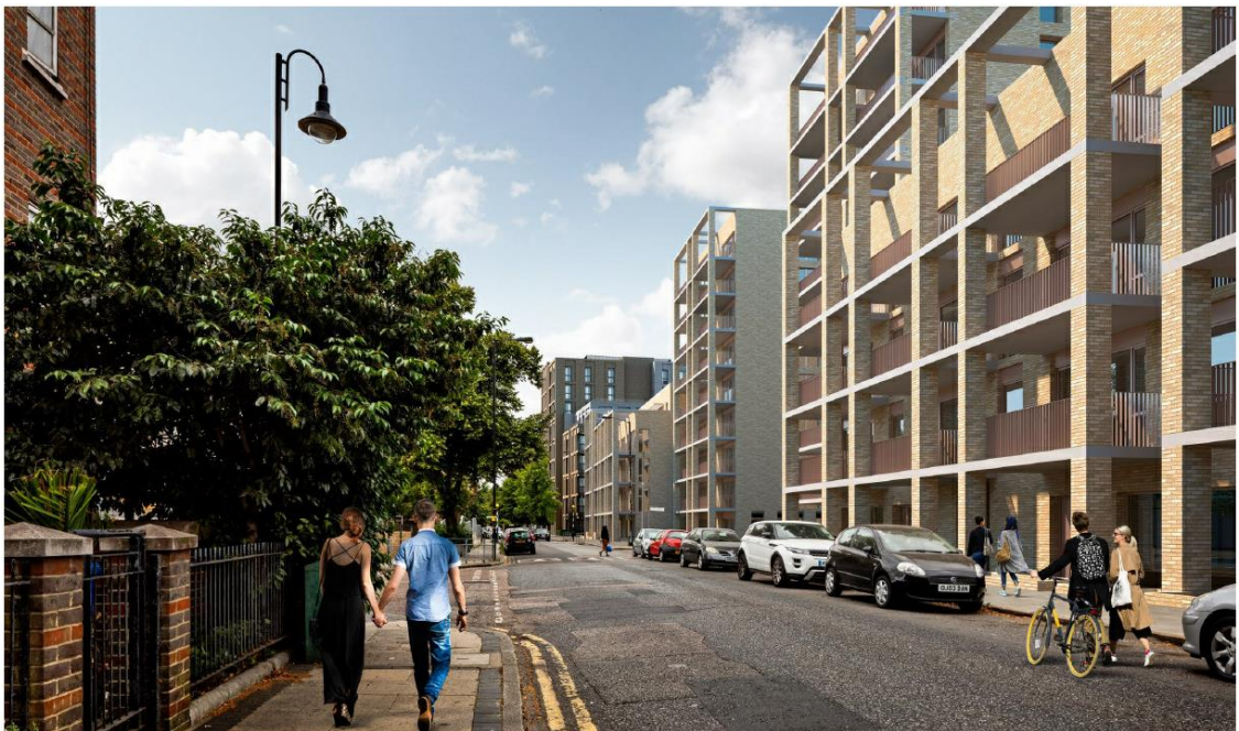
View from Commercial Way outside the approved and under construction 16/AP/4207 site looking east towards the application site. (Note: render reflects massing at initial submission)
