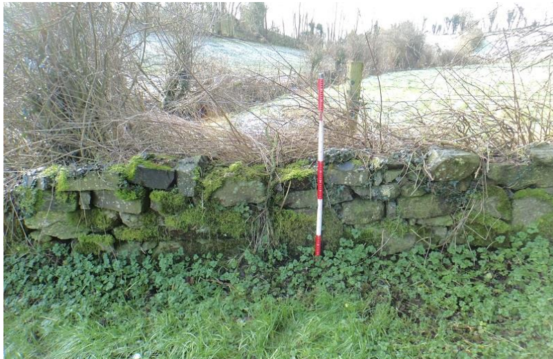
Plate 3 Graveyard boundary wall, facing west
