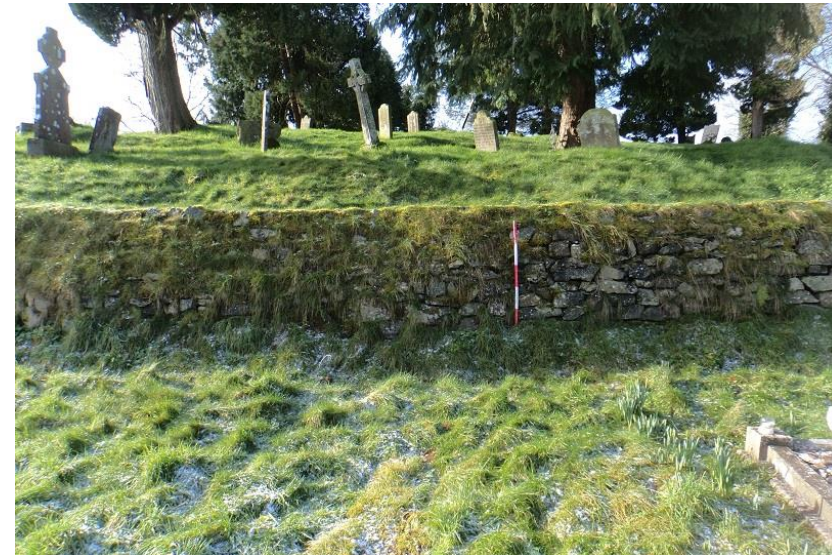
Plate 8 Retaining graveyard wall, facing southwest
