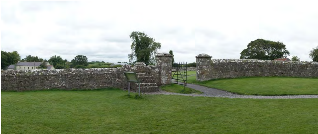
Plate 2-11. View from the bottom of the stairs on the south facing Façade.
