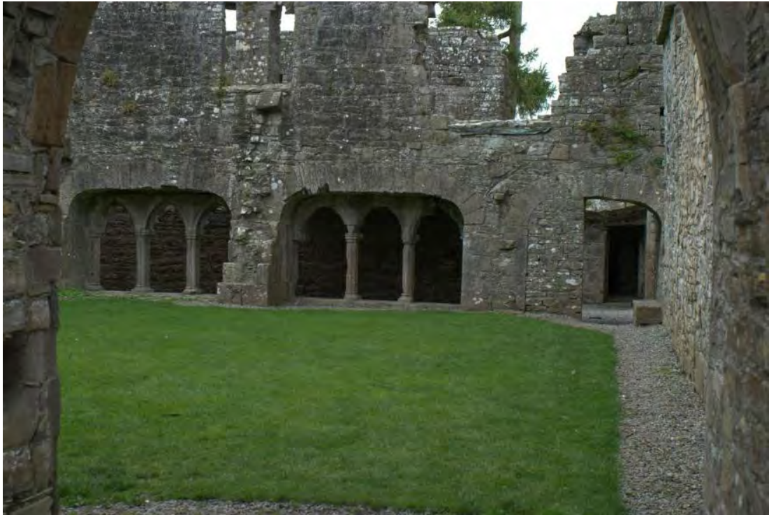
Plate 2-6. View into cloister.
