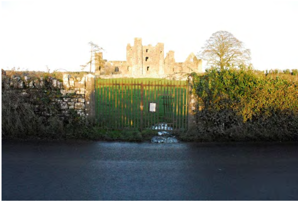
Plate 2-2. Previous access into Bective Abbey.
