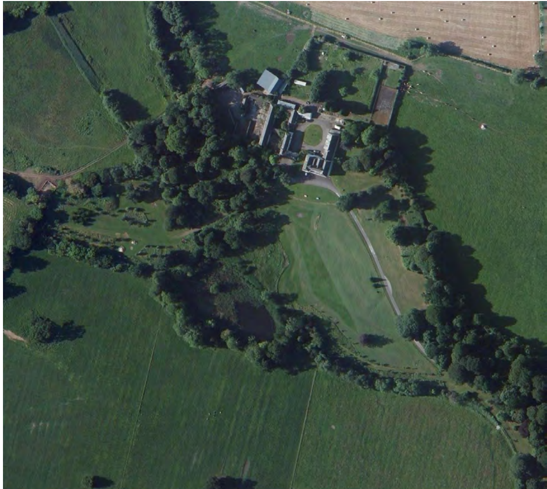
Figure 3-28. Detailed view of Dunderry Park (Philpotstown House) (Source: Bing Maps, accessed 12/10/2015).
