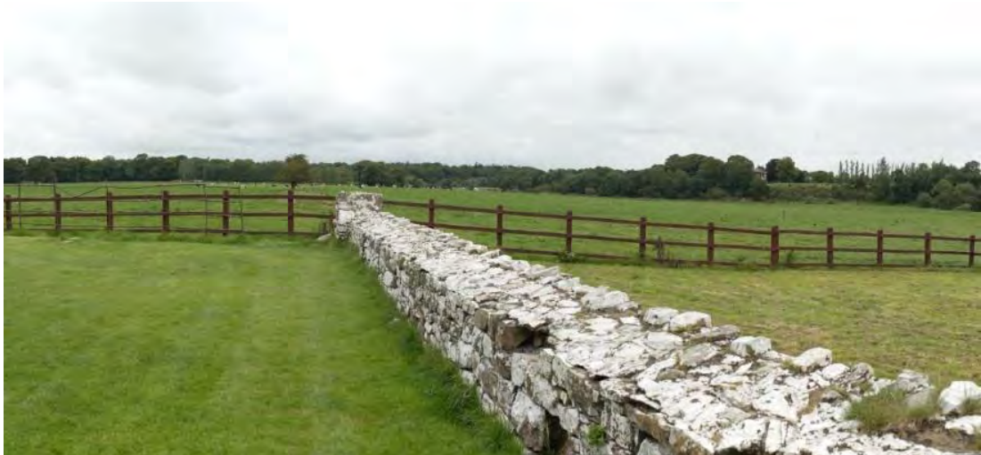
Plate 2-8. View north from nave towards the Boyne River and the Draft Tara Skryne LCA
