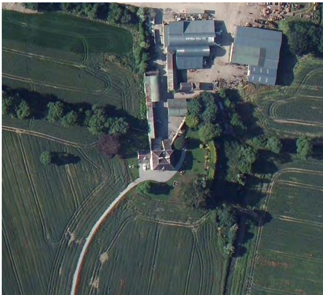
Figure 3-14. Detailed view of Churchtown House
