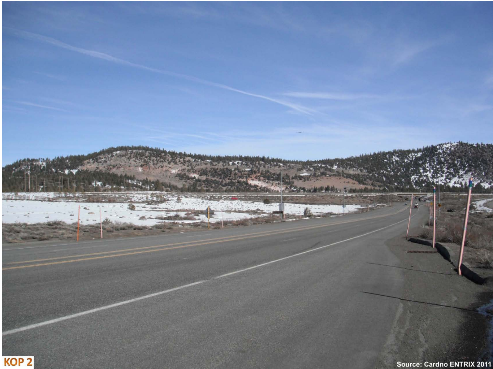
Figure 22: Existing View from Key Observation Point 2 (KOP 2)
