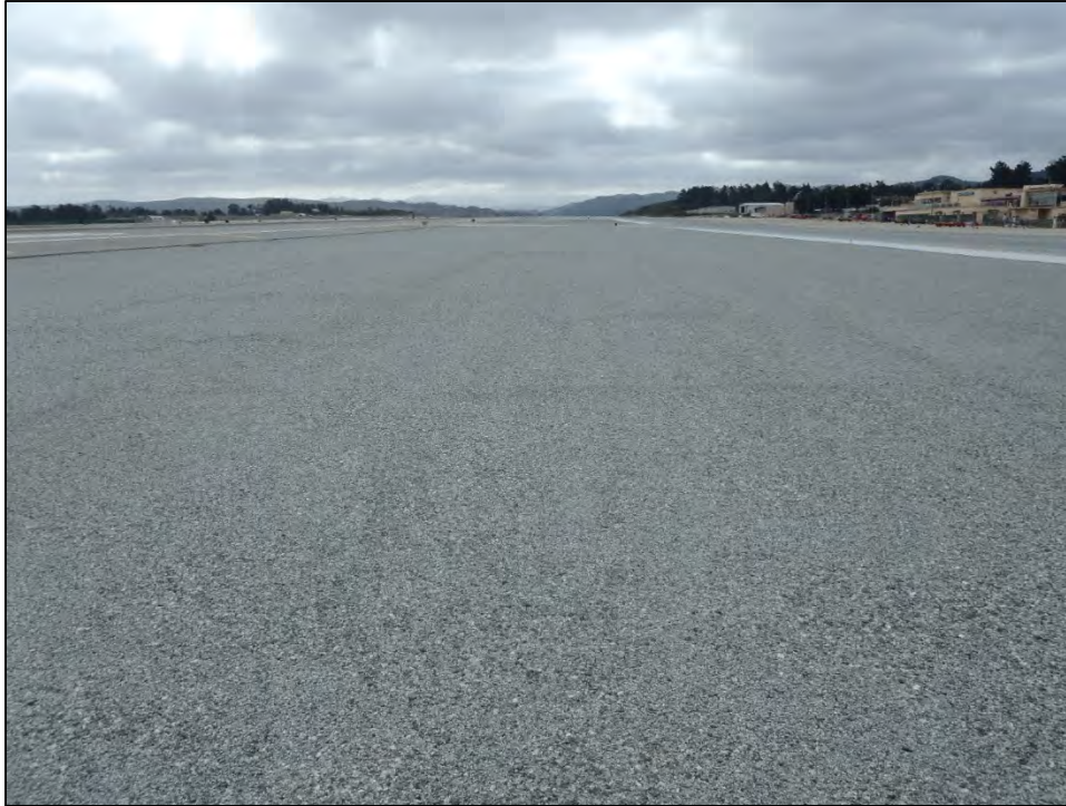
PHOTO 3: Representative view of the existing chipseal in the BSA.
