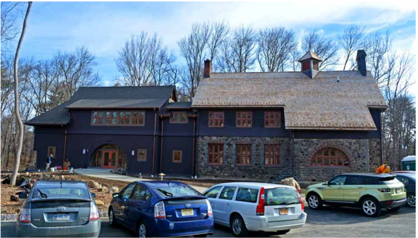
The view from the southeast side, showing new addition and original building in historically-matched paint scheme of 1891. The original 1891 bellcote over the front gable remains in situ without bell. The vented belfry was a later addition with bell intact and working by means of its pull-rope on the second floor landing. (Credit: NYNJTC)
