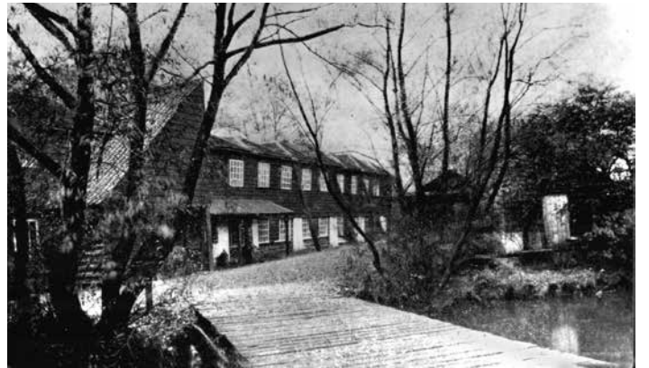
The dye house and stained-glass workshop looking across the bridge crossing the river Wandle. The stairs to the stained-glass workshop can be seen on the left of the photograph, c1898-99 (in L. F. Day, Art Journal ).
