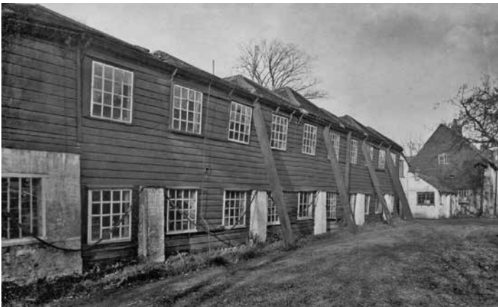
The dye house on the ground floor with the stained-glass workshop above. At the far end of the stained-glass workshop was the original location of the tapestry workshop, 1913.
