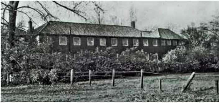
The carpet and block-printing workshops from the bleaching fields. In front of the building are the gardens where the workers could grow vegetables and flowers, 1913.
