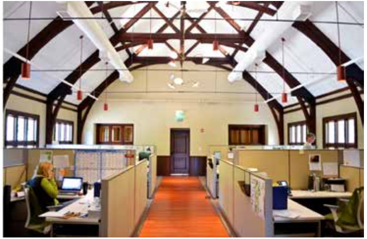
The unrestored and restored community hall on the upper level. Original windows on the end-wall are now display cases. New HVAC ductwork hangs from cables. The door at the far-end leads into the new addition. (Credit: NYNJTC)
