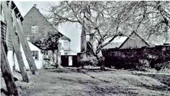
Looking towards the entrance to the works with the 18th-century caretaker's house and the little office on the left, early 20th century.
