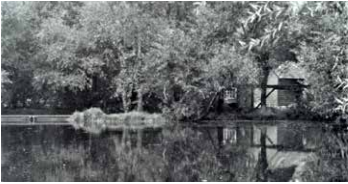
The boiler house, looking over the mill pond, early 20th century.
