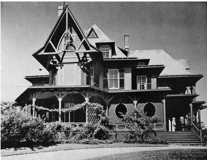
Figure 1: The Jacob Cram House of 1872, architect Dudley Newton’s “modern gothic” vernacular in wood, according to Vincent Scully, the stick equivalent of Philip Webb’s brick Red House. (Credit: Scully)
