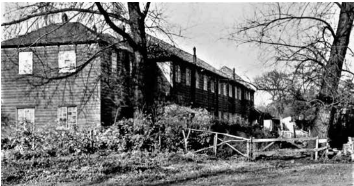
The rear of the carpet and block-printing workshops, 1913.
