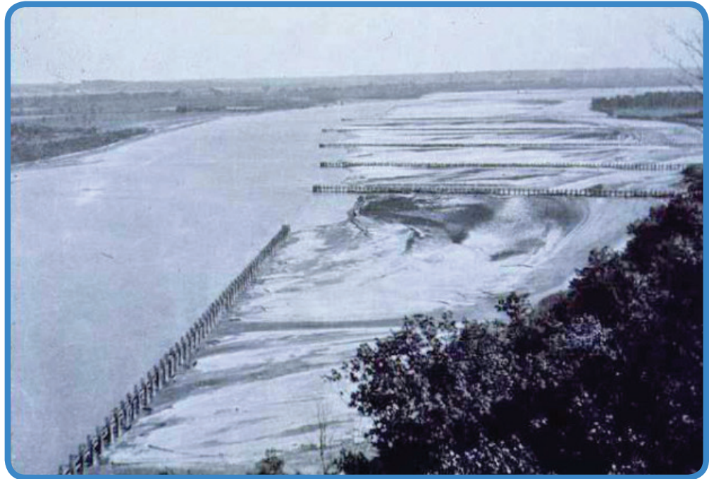
This is the Missouri River at Indian Cave Bend one year after channelization began, in October 1935.
