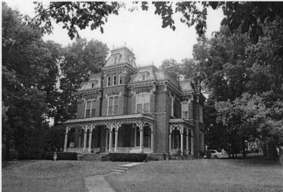
Figure Seven: A. F. Davis House, 301 West Spring Street
