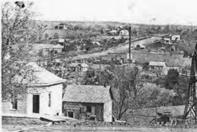
The city windmill at the right and the city power plant at the rear are shown in the 1890 photograph. The large house at the left in the distance was the John Cummings home.
