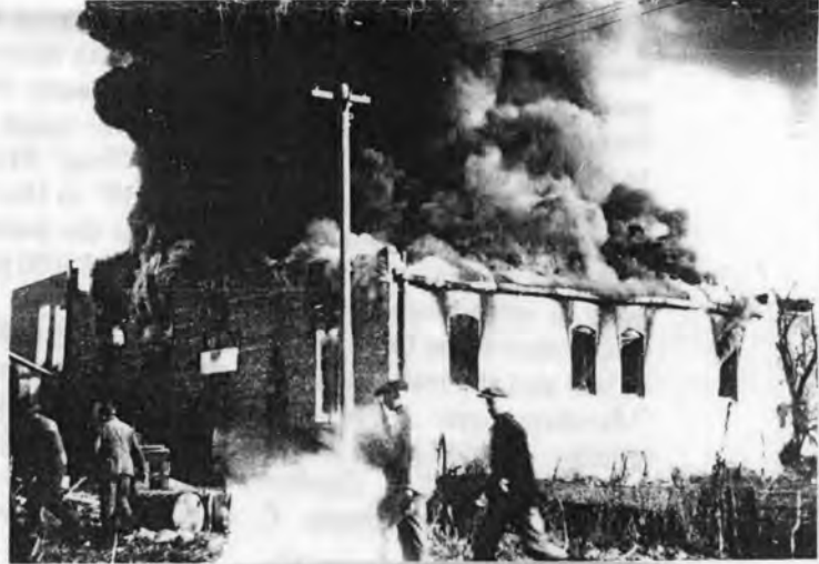
The Theatre Building was built in 1918 and burned in 1925. Haينه Restaurant in east side when it burnt.
