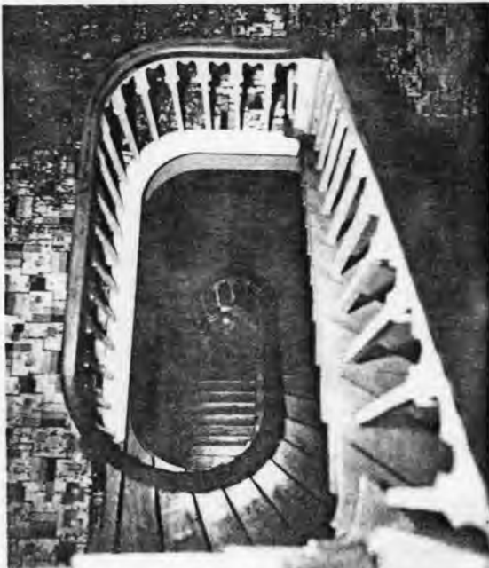
View looking down on the winding stairway that serves three floors of the Krueger Building in Washington.
