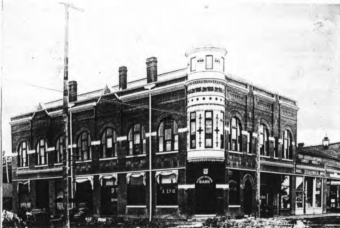
The Citizens National Bank with the Opera House on the upper floor. Note the elaborate trim and the steel roll shades to protect the large windows.
