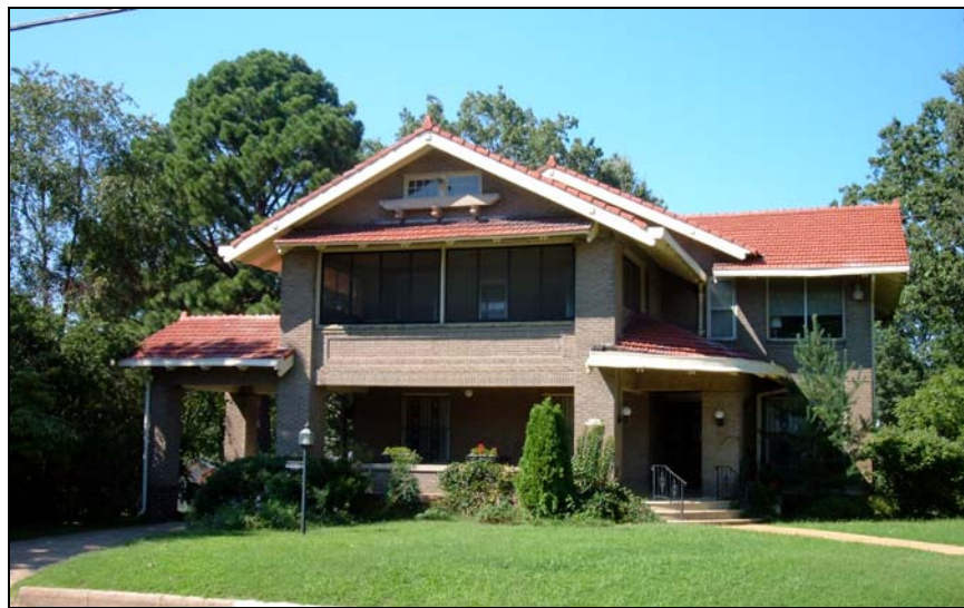
The Greer House at 955 Kinzer Street is a notable example of the Craftsman style (NR).
