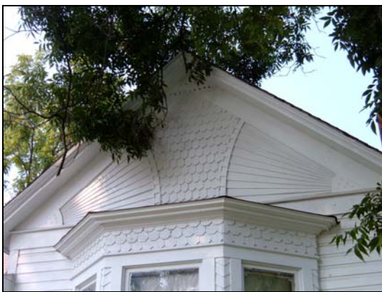
Fish scale shingles and sunburst panels at 305 N. B Street.
