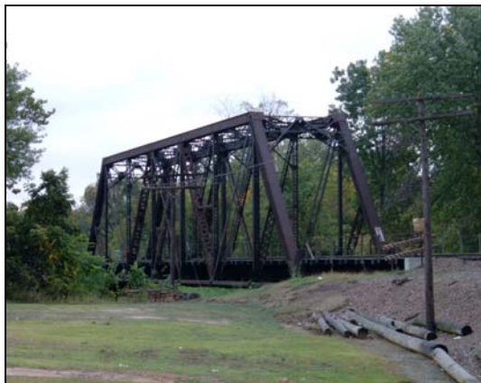
The Missouri Pacific Railroad Bridge.
