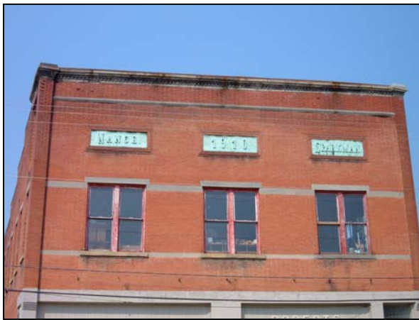
Upper façade of 313-315 N. Broadway.
