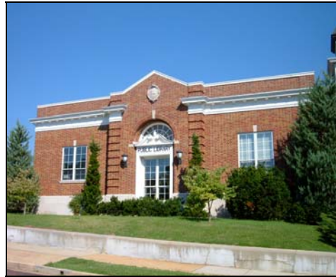
The original section of the Public Library (NR).
