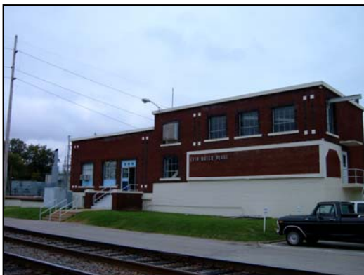
The City Water Plant.
