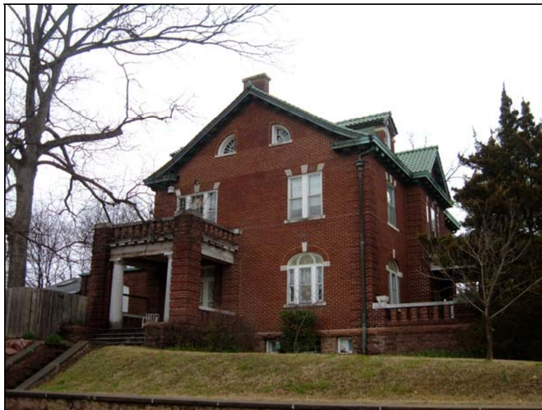
The John C. Corrigan House at 225 South Sixth Street is an excellent example of the Colonial Revival style (NR).
