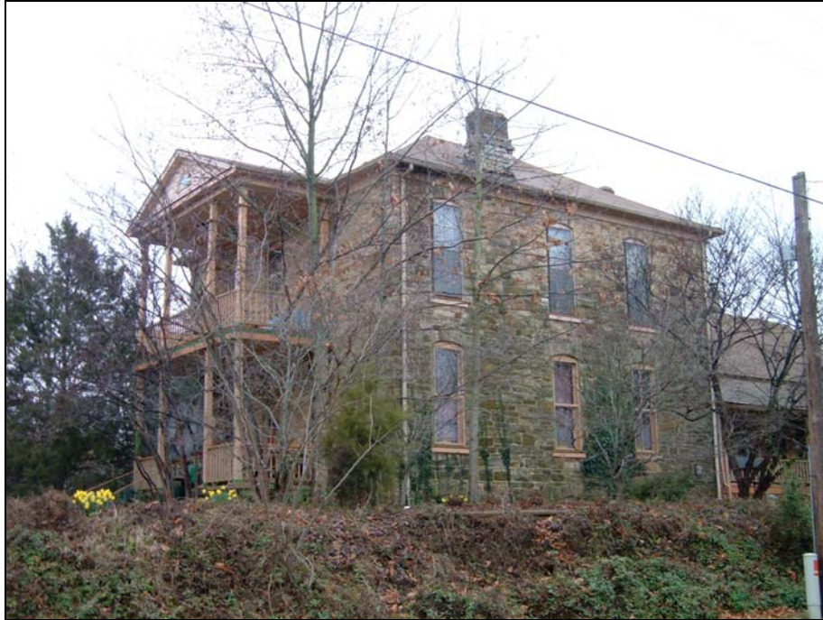
The Luke F. Quinn House at 303 South Sixth Street (NR). This Italianate style dwelling is of stone construction and features segmental arched windows and a hipped roof.
