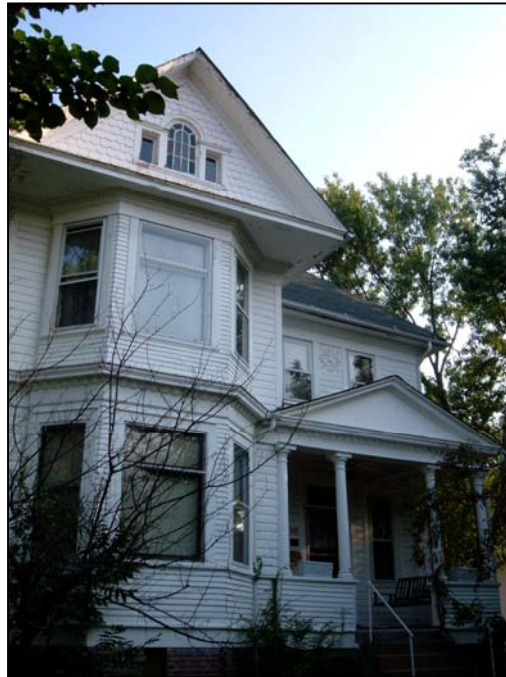
The Thomas Moore House at 435 Lester Street is an example of a Queen Anne/Colonial Revival style dwelling. It has an asymmetrical form and classical porch columns (NR).
