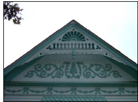
Gable detailing at 723 9 th Street.
