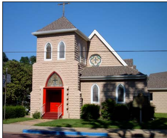
Holy Cross Episcopal Church was built in the Gothic Revival style.
