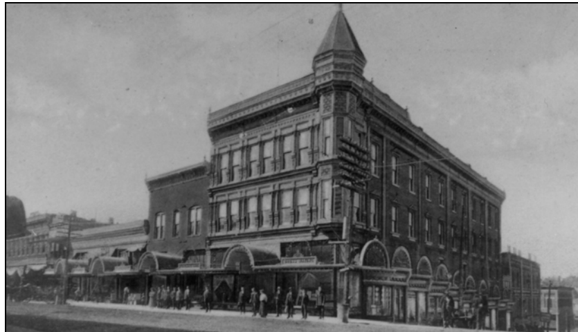
The large Wright-Dalton-Bell-Anchor Department Store at the corner of Main and Poplar Streets. (Photo courtesy of Bill Hogg)
