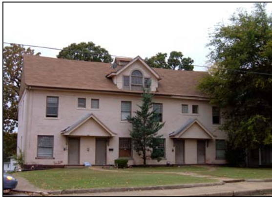
Colonial Revival style apartments at 445-447 N. Main Street.
