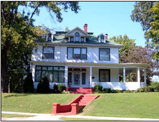
Colonial Revival style Bacon House at 808 N. Main Street.
