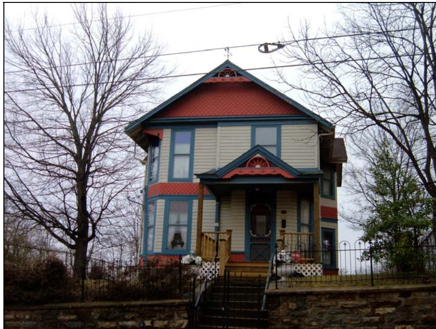
The John Archibald Phillips House at 522 Cherry Street is a notable example of the Queen Anne style. This style features an asymmetrical form, eave vergeboard, and decorative woodwork (NR).
