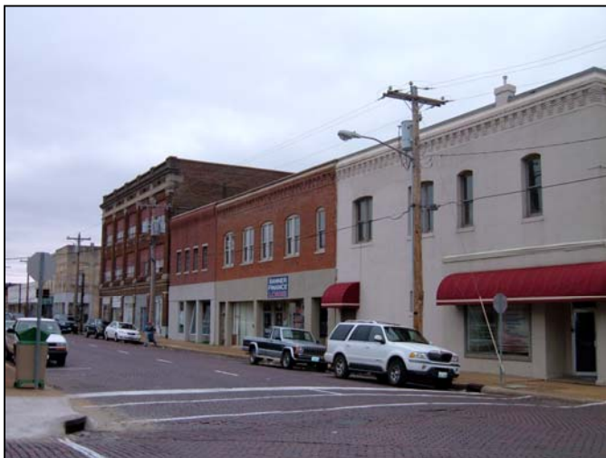
Several historic commercial buildings are located on S. Broadway (NR).
