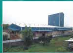
Feed Plant - Gujarat
