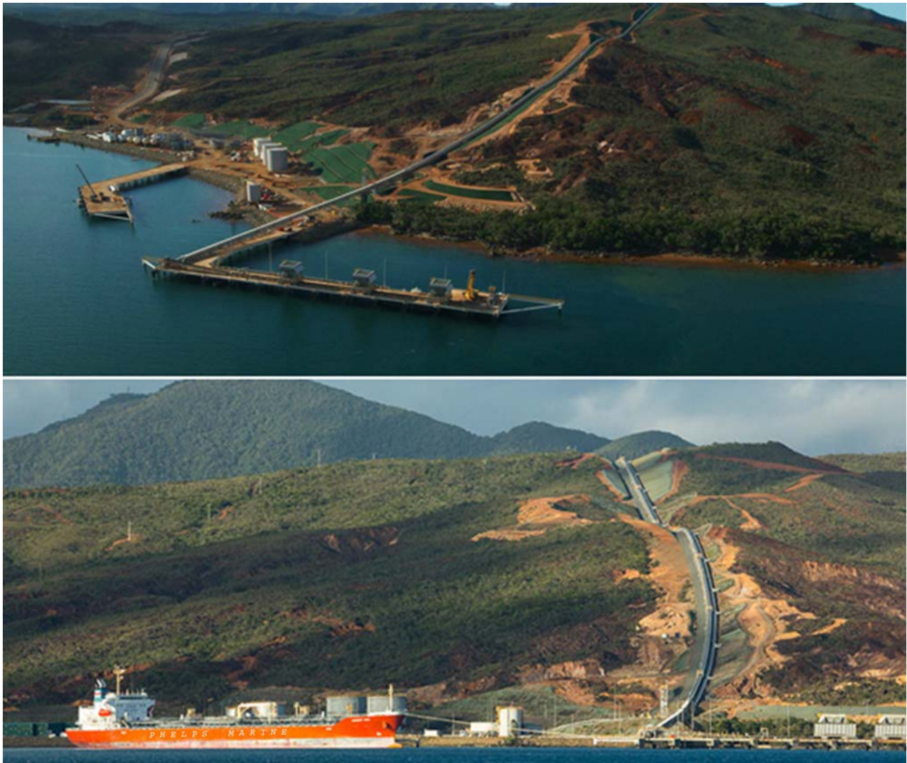
Port of Prony Nickel Ore Quay
