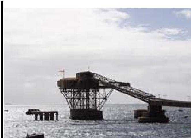
Rade de Thio Ore Loading Berth
