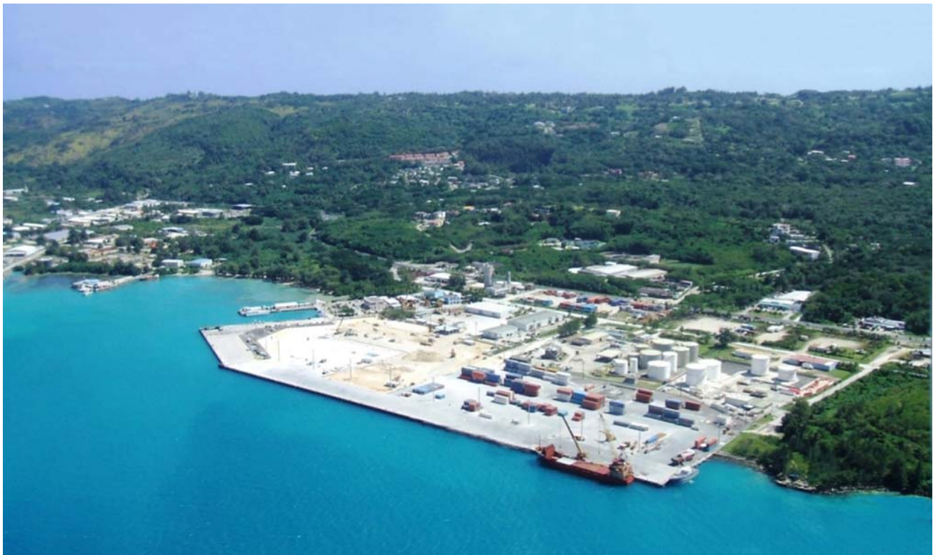
Saipan—Puerto Rico Wharf
