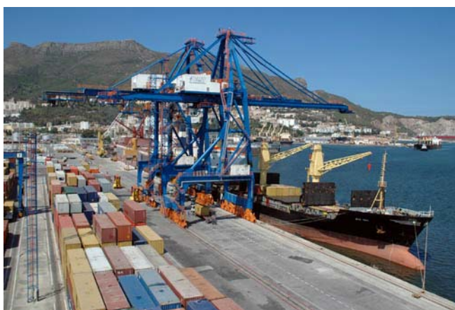
Oran Container Pier
