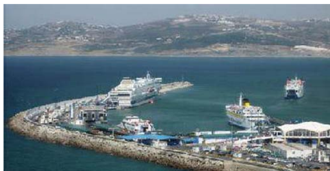
Port of Tanger Breakwater from W
