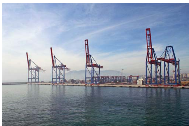
Wharf 9—Container Terminal
