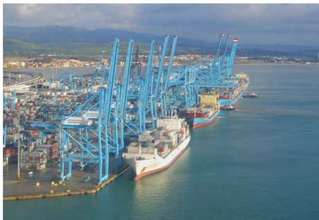
Maersk Container Terminal
