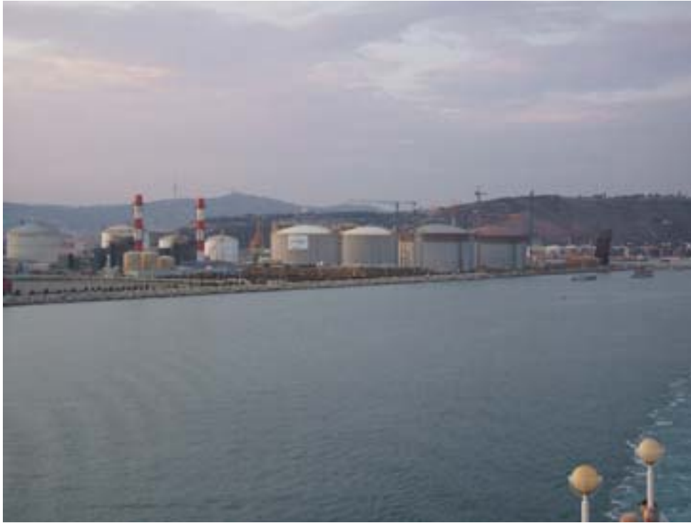
Barcelona—Tanks and stacks S of Harbor Control Tower
