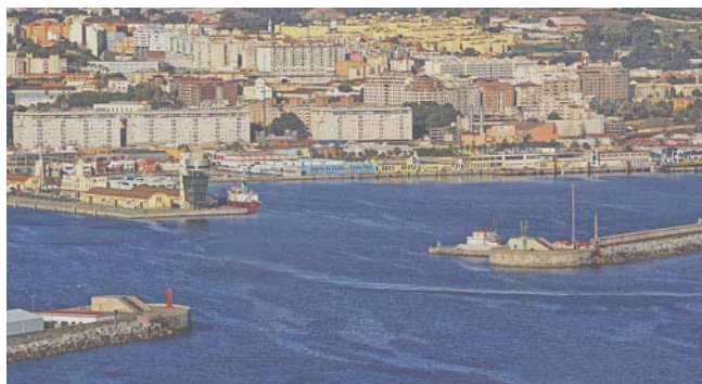
Ceuta Harbor Entrance
