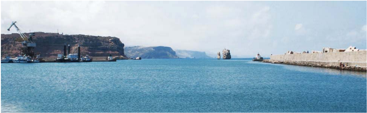
Ghazaouet Breakwater and Les Deux Freres in distance
