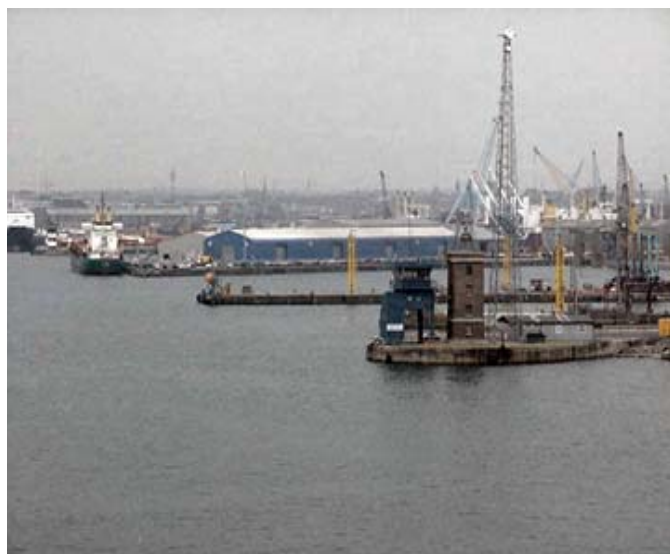
Courtesy of USCGC CAMPBELL Dublin—Port Radio/Radar Station
