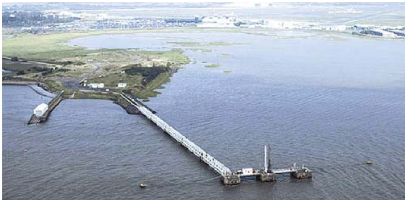
Shannon Airport Oil Jetty
