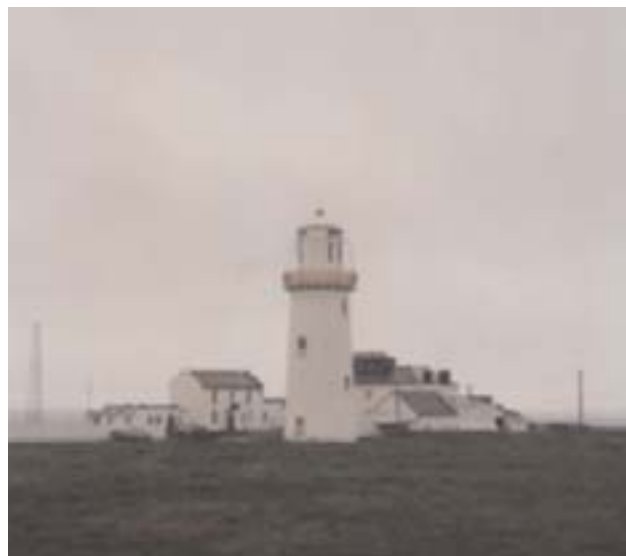
Courtesy of the Commissioners of Irish Lights Loop Head Light
