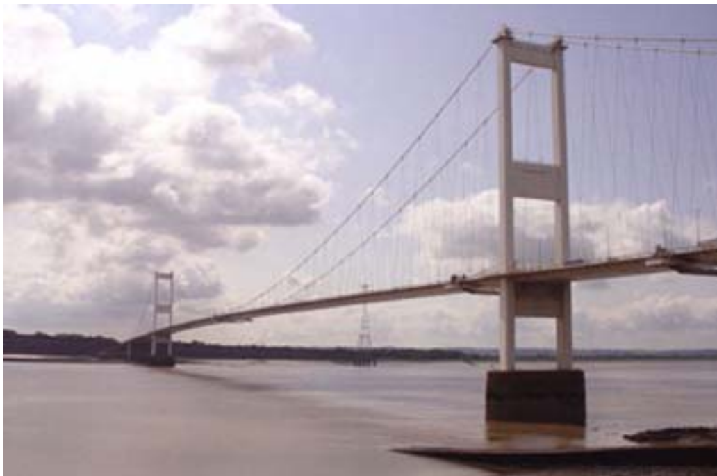
The Severn Bridge
