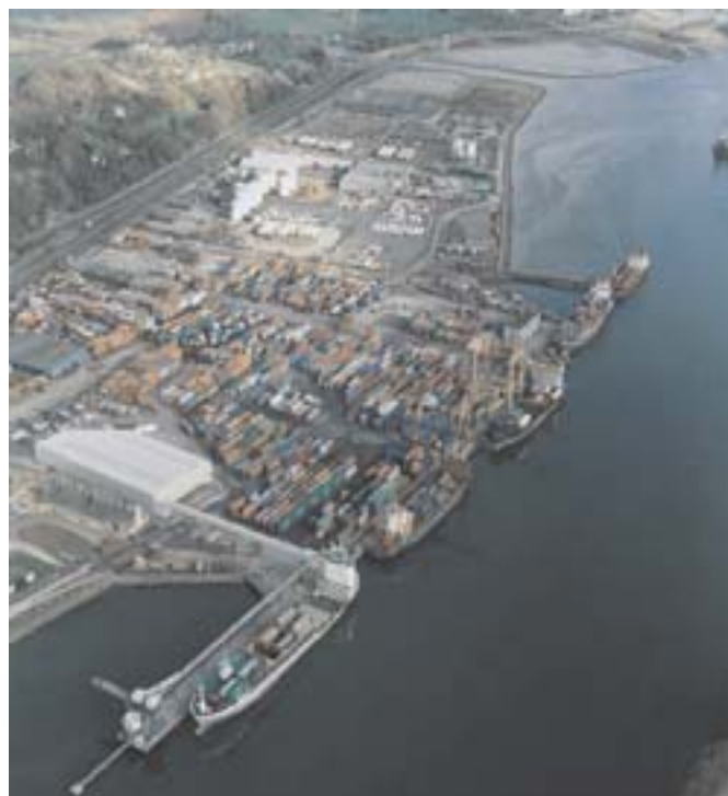
Cork—Tivoli Container Terminal
