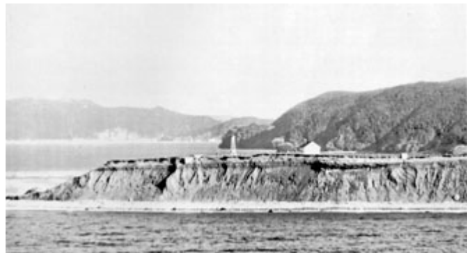
Point Verde Light—approach (replaced by skeletal tower)
