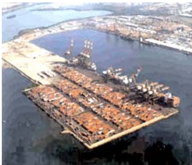
Gordon Cay (South Container Terminal)
