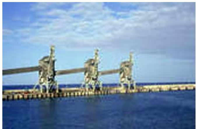
Bridgetown—Conspicuous Sugar-loading Towers
