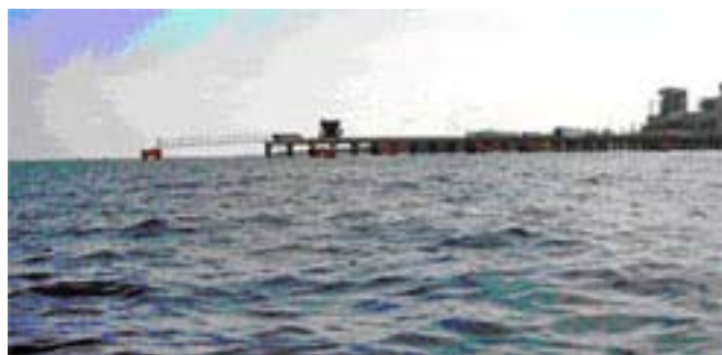
Puerto de Haina—ITABO Fuel Pier
