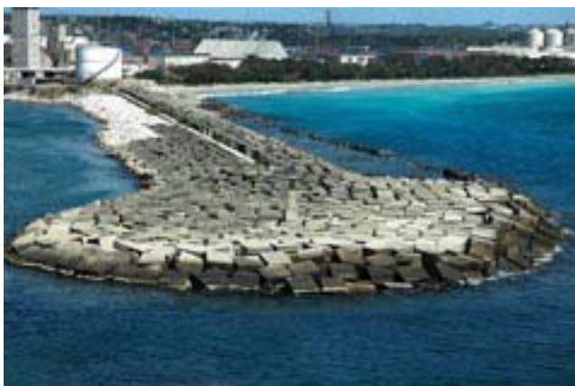
Puerto de Haina—East Breakwater Light
