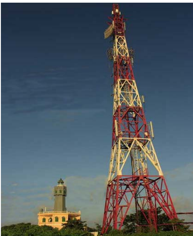
Bach Long Vi Lighthouse beside a communication tower
