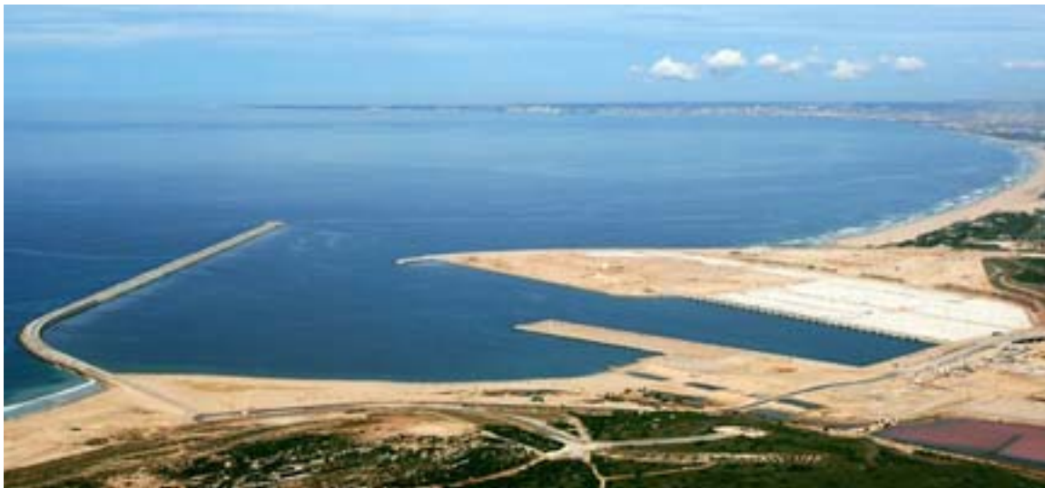
Port Ngqura—Aerial view
