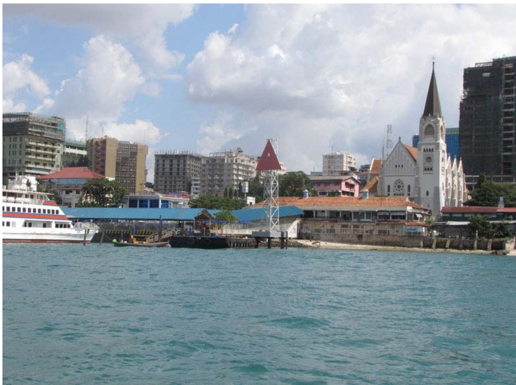
Dar es Salaam Harbor—Passenger Pontoon Pier
