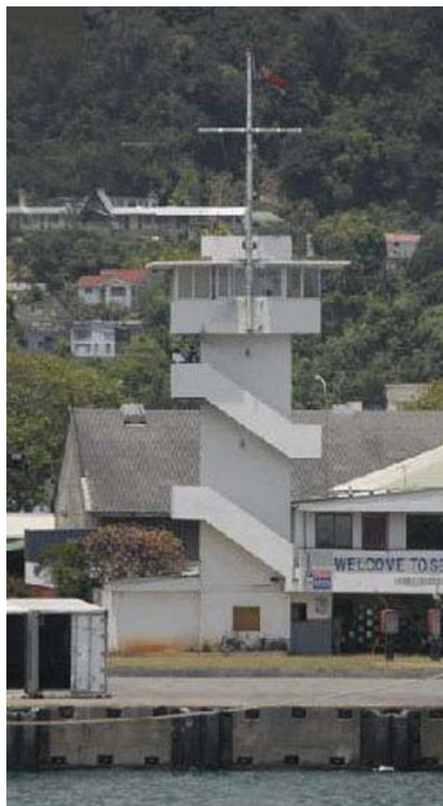
Port Victoria Control Tower/Signal Station
