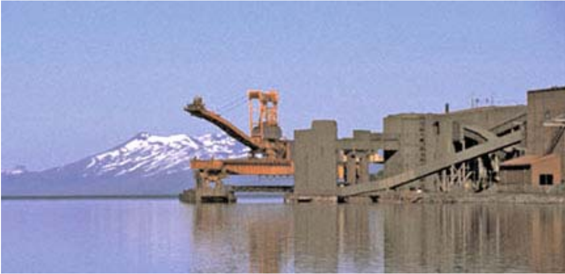
Narvik—Iron Ore Terminal
