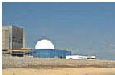
Sizewell Nuclear Power Station
