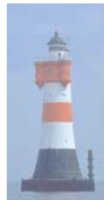
Roter Sand Tower
