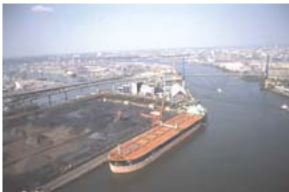
Hamburg Bulk Terminal
