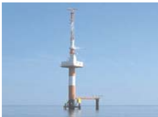
Hooksielplate Radar Tower
