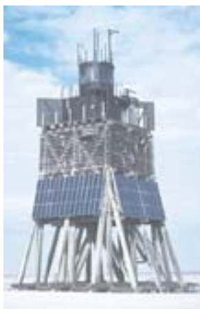
Suderoogsand Light (Refuge Beacon)
