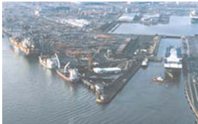
Bremerhaven—Nordschleuse (North Lock)
