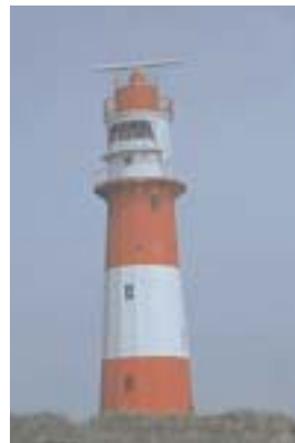
Borkum Little Disused Light Tower
