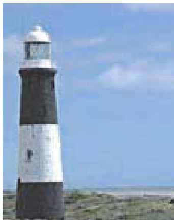
Spurn Head Lighthouse (disused)
