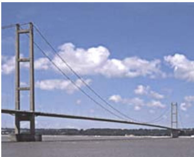
The Humber Bridge
