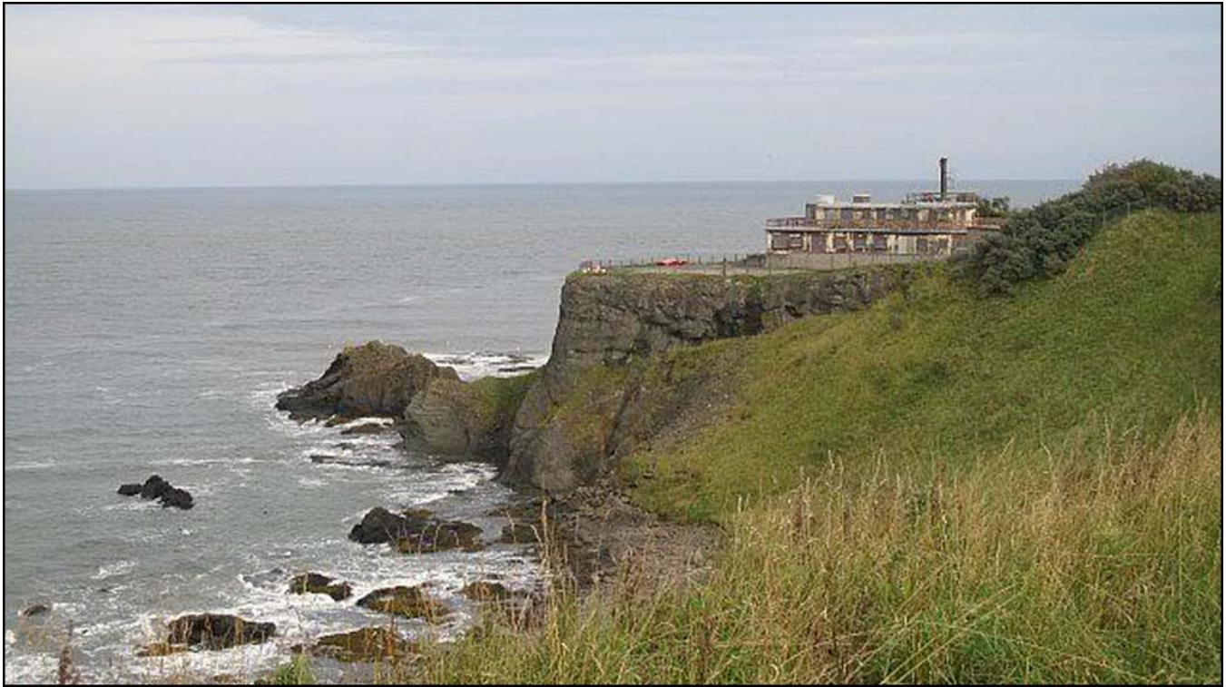
Ginhead—Stack and Buildings
