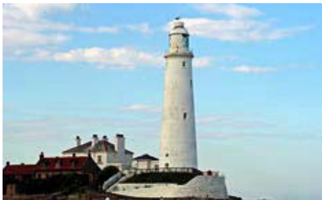
St. Mary's Island Disused Lighthouse
