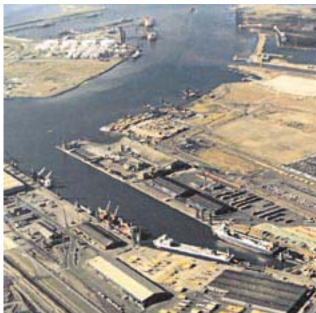
Tees Dock and Norseia Oil Terminal
