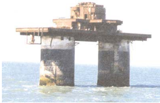
Knock John Tower
