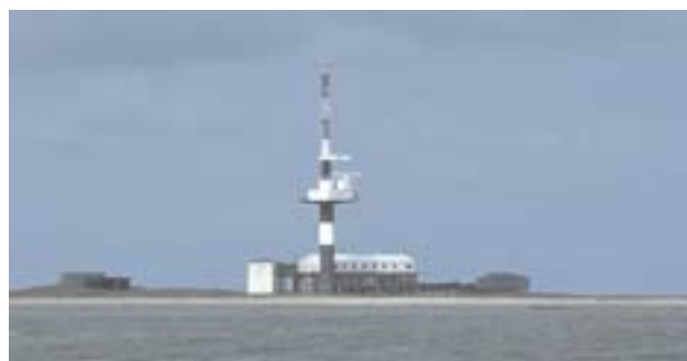
Oldoog Radar Tower (Minsener Oog Buhne C)
