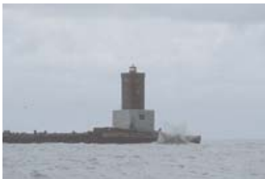
Minsener Oog Disused Light Tower (Buhne A)
