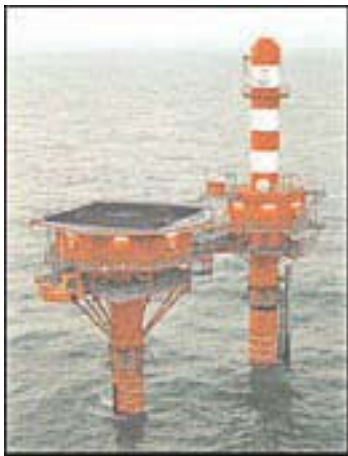
Oostdyck Radar Tower
