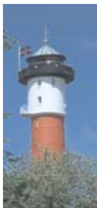
Wangerooge Disused Light Tower
