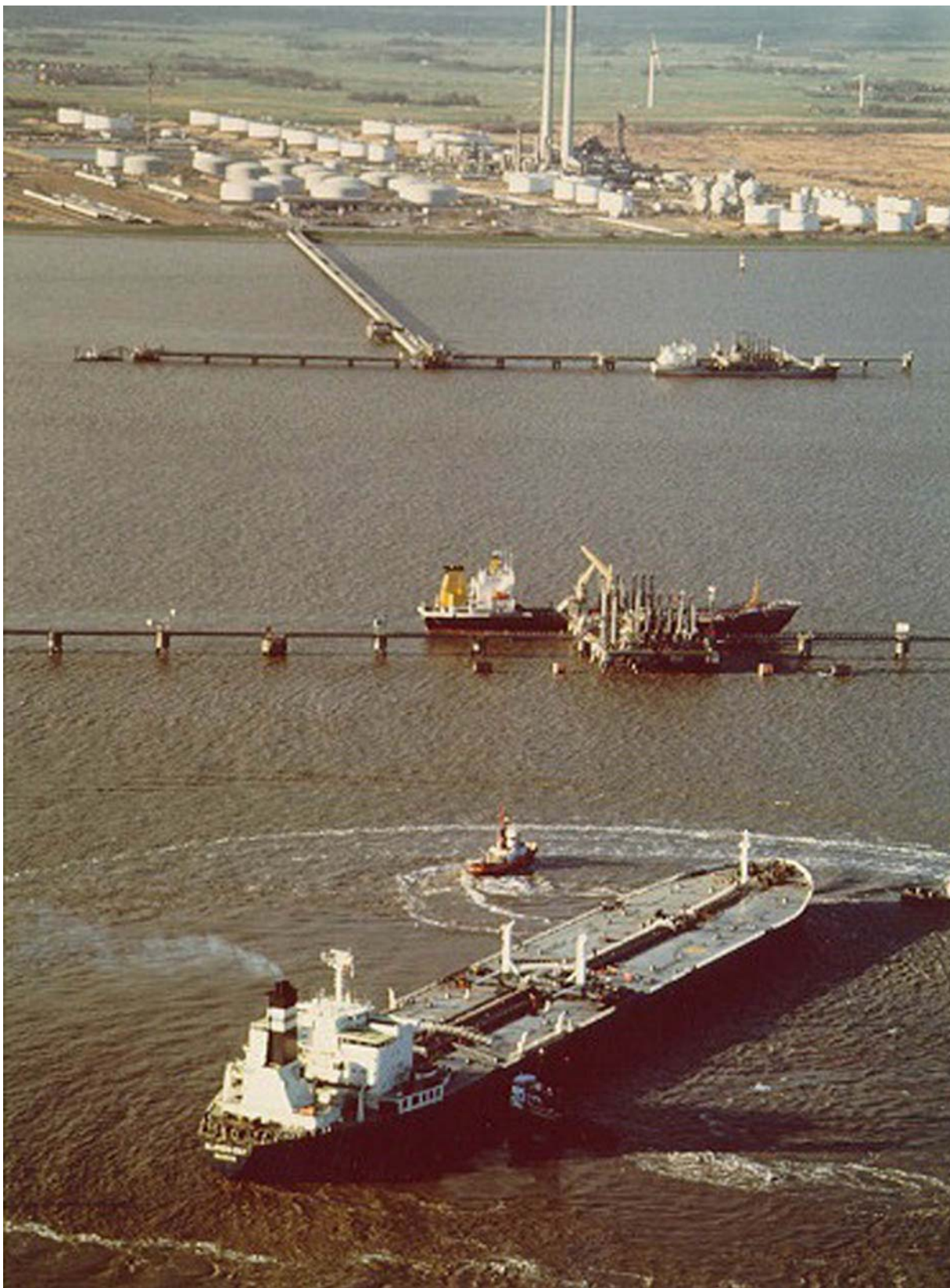
Wilhelms WRG Terminal
