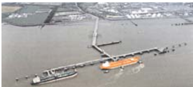
Immingham Oil Terminal
