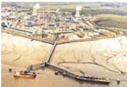
Salt End Oil Terminal
