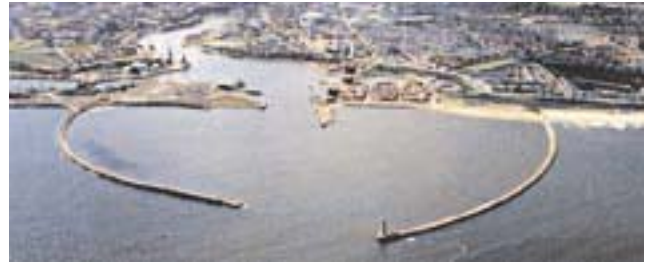
Entrance to the River Wear (Sunderland)
