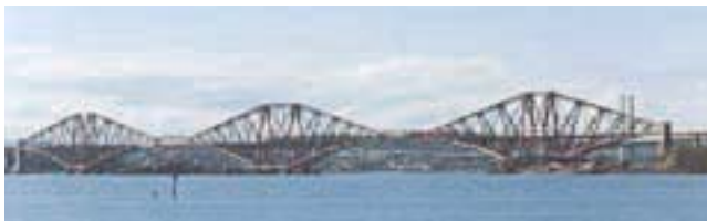
The Forth Bridges from NE
