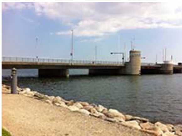
The Hadsund Bridge
