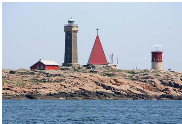
Vinga Light, day beacon, and radar tower
