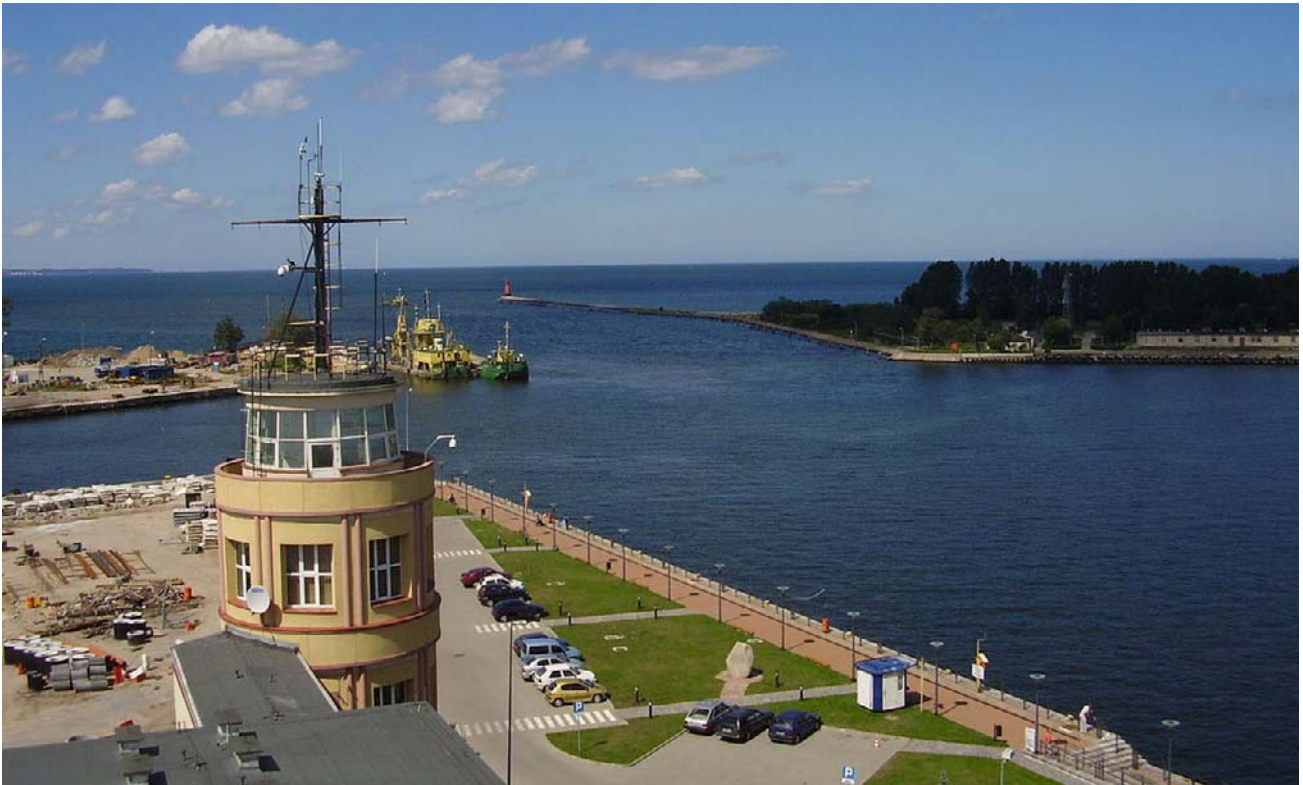
By Pazurzasty [CC-BY-SA-3.0 ( https://creativecommons.org/licenses/by-sa/3.0 )], from Wikimedia Commons Gdansk Harbor Entrance—Port Office Building as viewed from the old lighthouse
