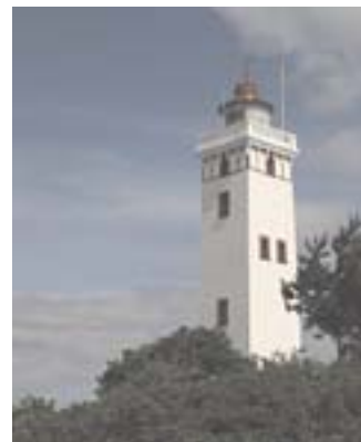
Strib Light (Strib Odde Light)
