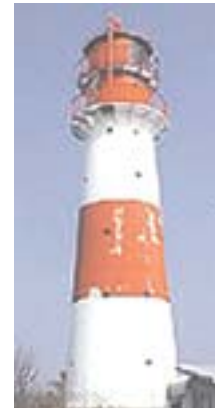
Falshoft Disused Light Tower
