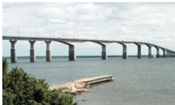
The Olands Bridge
