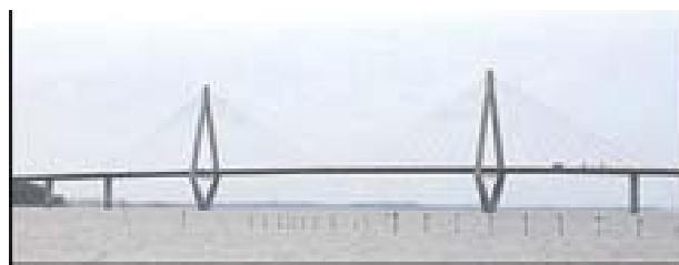
The Faro Falster Bridge
