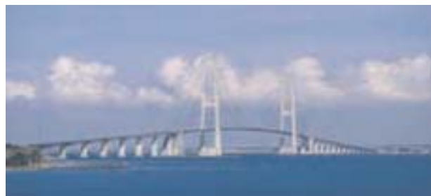
Store Baelt Link—East Bridge
