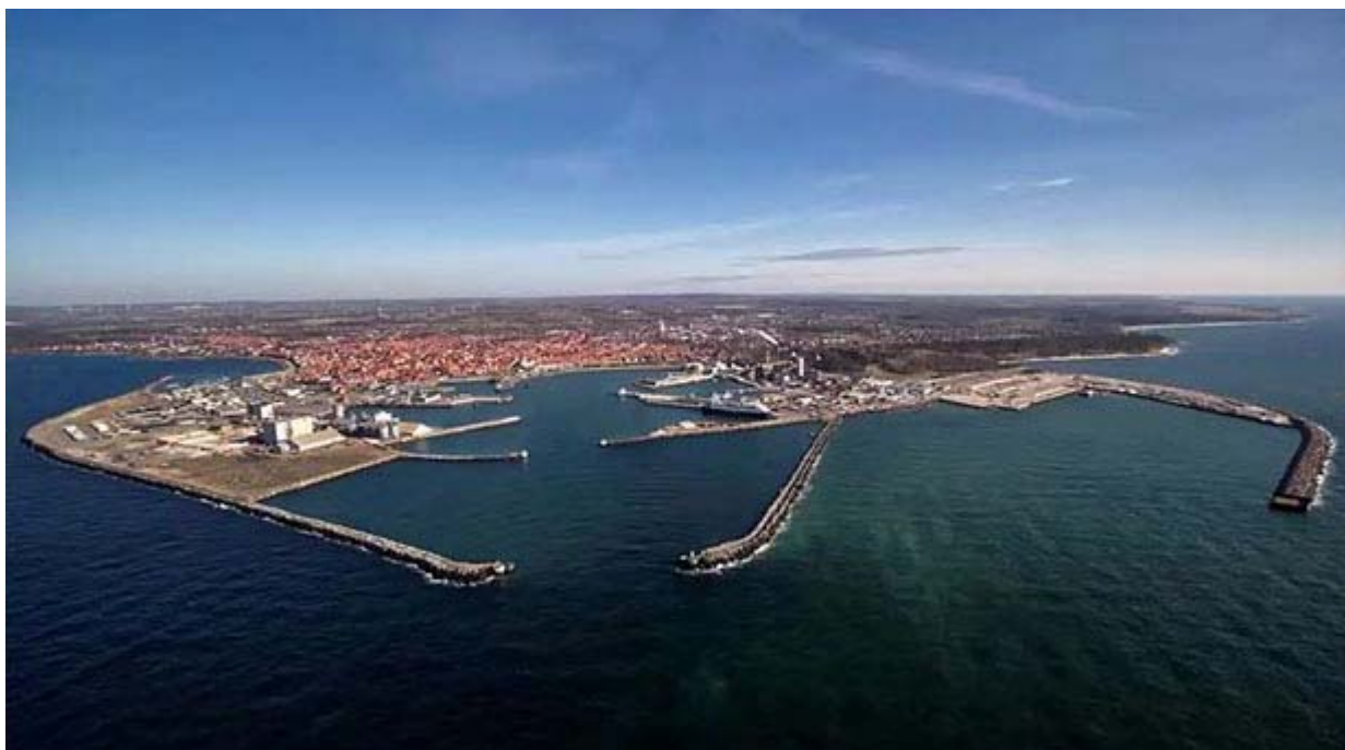
Ronne Havn A/S - Commercial Port of Bornholm https://www.roennehavn.dk/en/port-expansion/drone-photos/
