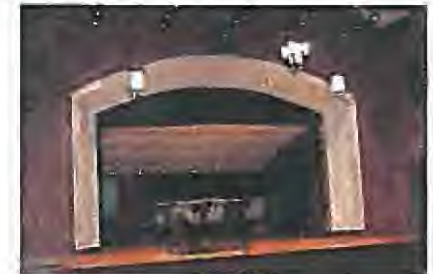
Fire sprinklers in Akin Auditorium
