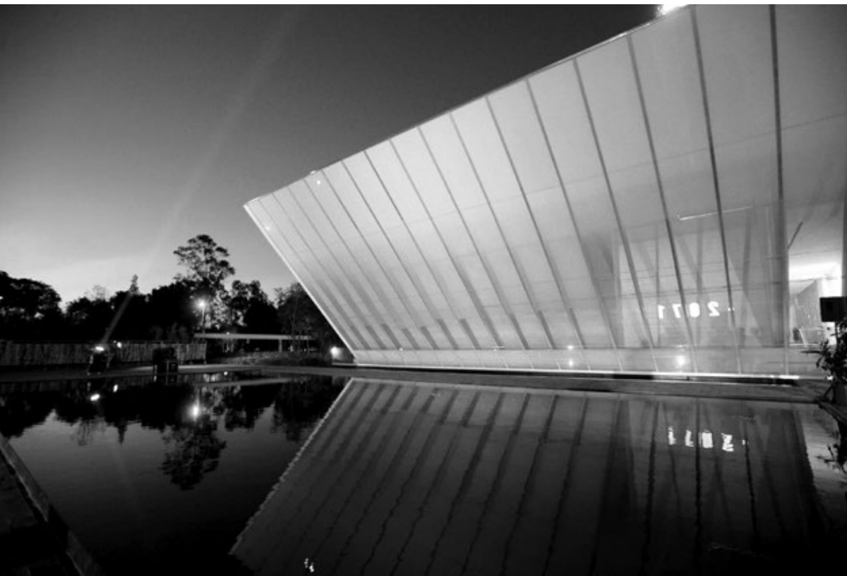
Vista frontal del—Facade view from the Museo Universitario Arte Contemporáneo, MUAC, 2008. Foto—Photo: Barry Domínguez
