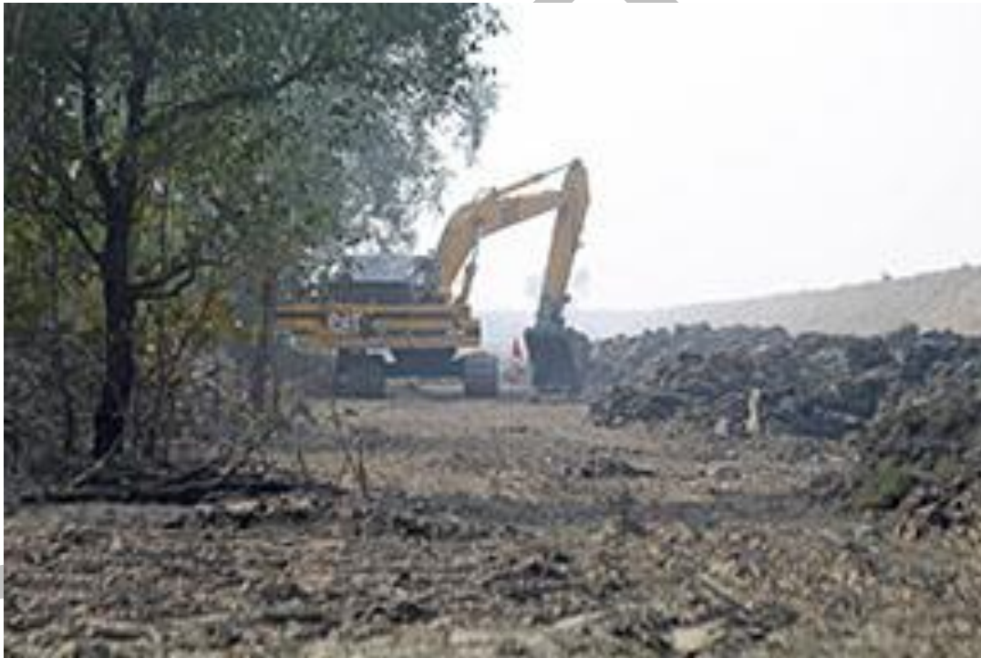
Construction of road in coastal mangroves.
