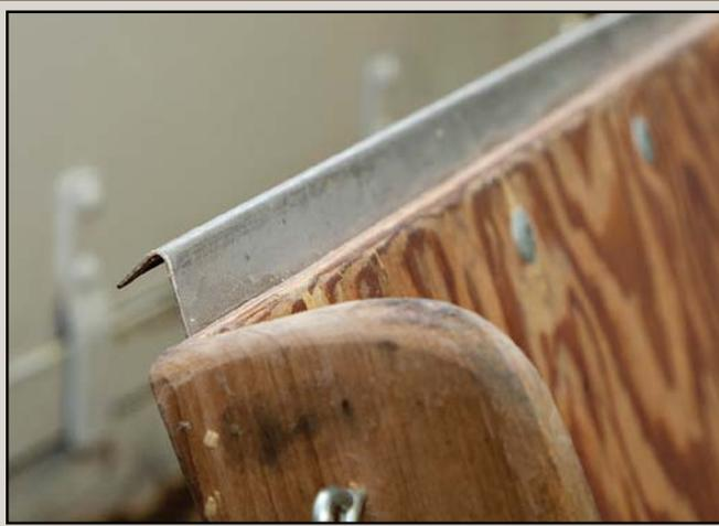
FIG. 3. Metal lip used to attach slide to steel track of exhibit.
