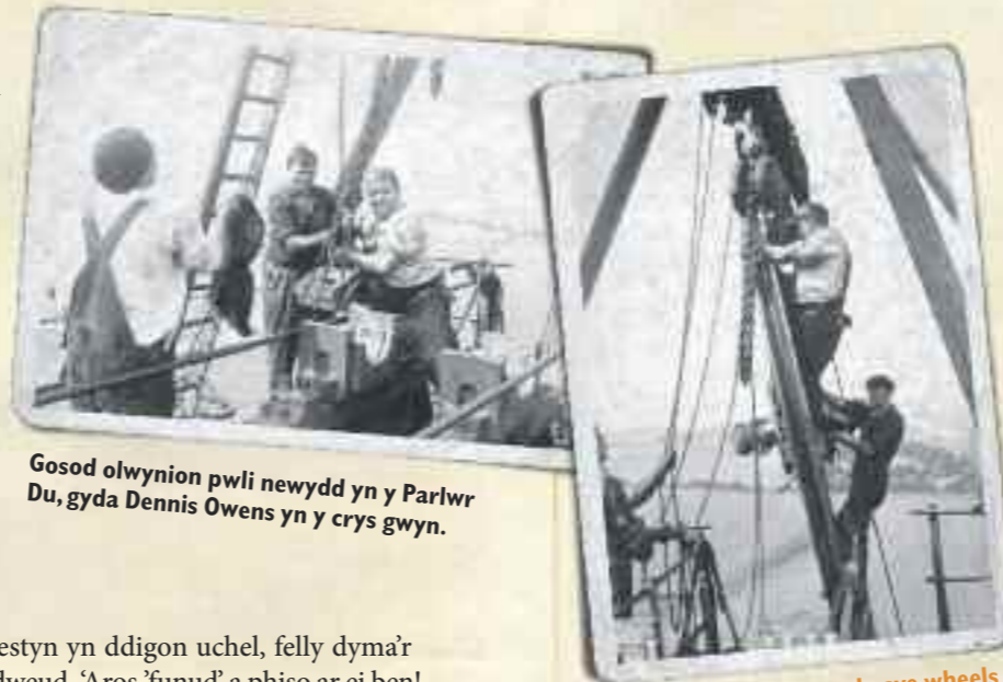
Installing new sheave wheels at Point of Ayr Colliery, Dennis Owens in white shirt
