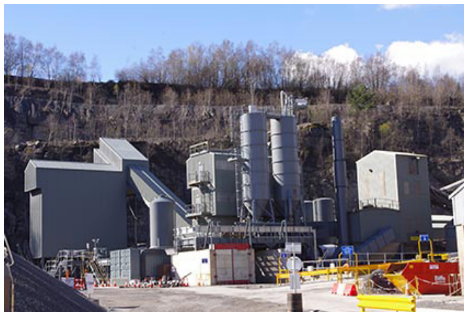
Fig.1 Processing plant, Craig y Hesg Quarry
