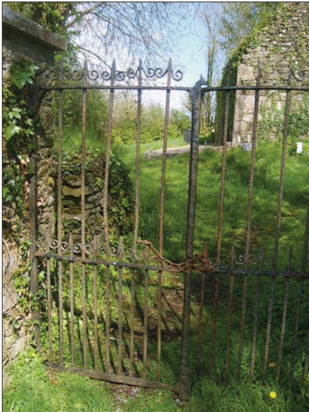
PLATE IV. A wrought iron gate at Kilbonane, probably late nineteenth to early twentieth century, is located in the entrance way at the western end of the graveyard. This metalwork could do with some cleaning and paintwork, and repair, otherwise it will fast deteriorate, and portions of it will fall off
