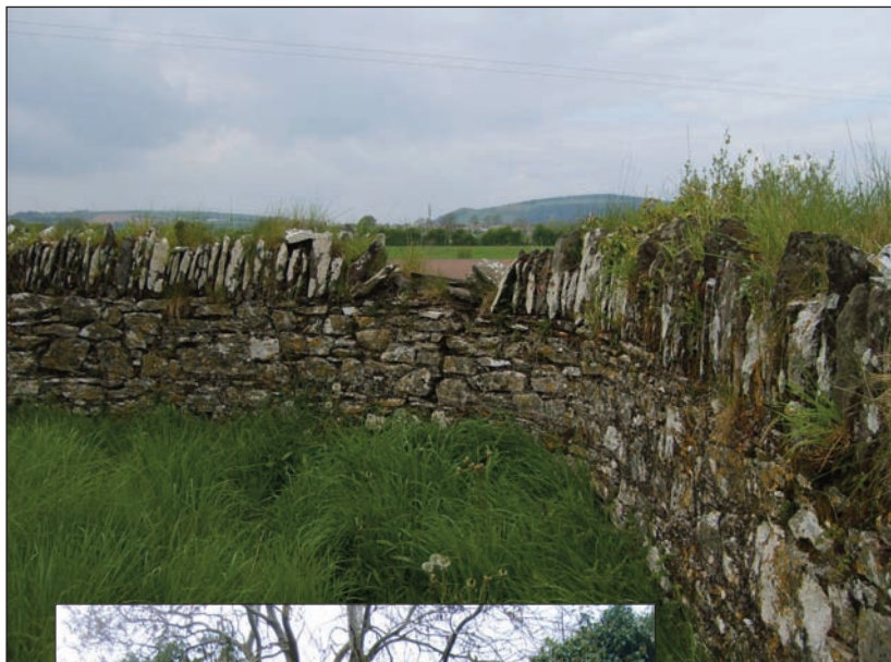
▼ PLATE XII. The perimeter walling around Kilnaglory church and graveyard. A large vertical crack is evident at the bend of this walling and immediately above it, the vertical cap stones are missing
