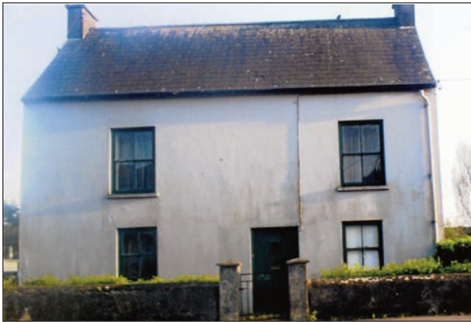
Former Ballincollig Courthouse, near the East Gate
