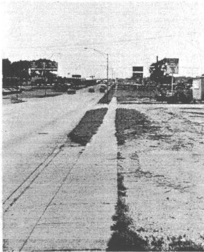
FIGURE 14. PHOTOGRAPHS OF THE WEST "O" ST. SAFETY IMPROVEMENT PROJECT.
