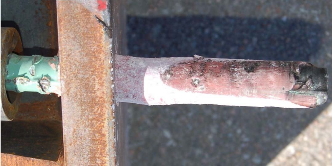
Figure 56. Post-Test Anchor Photograph, Test No. WEAB-11
