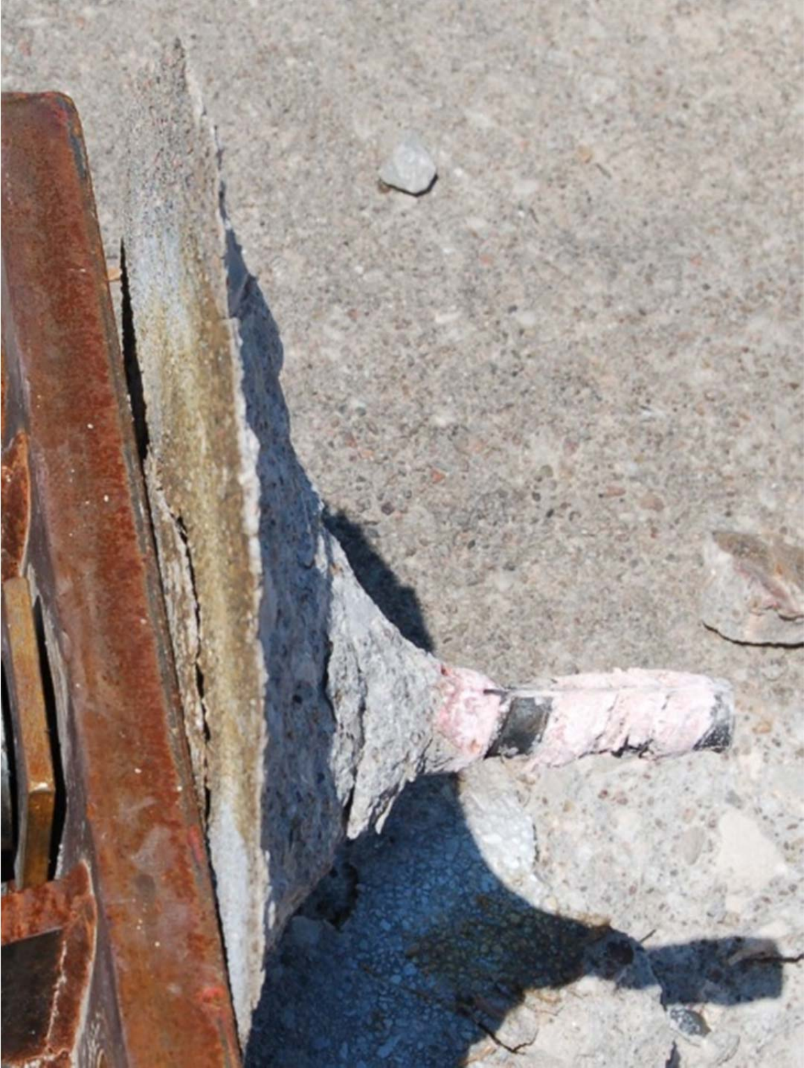
Figure 82. Post-Test Anchor Photograph, Test No. WEAB-17
