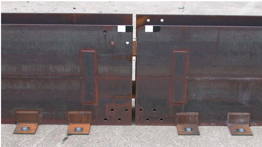
Figure 7. Steel H-Section Temporary Barrier Anchors
