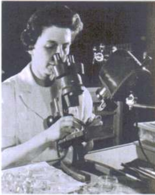
Microscopic inspection of precision quartz crystals assure high quality and performance for defense and industry needs.
