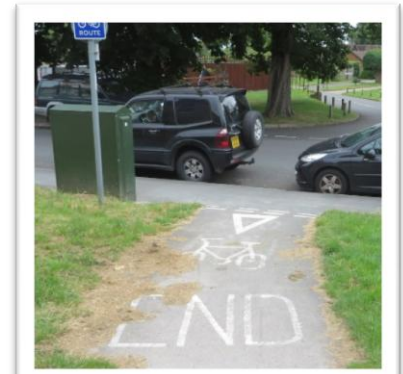
French Street, leaving path "TP26" Road markings used in conjunction with the 'End of Route' signing
