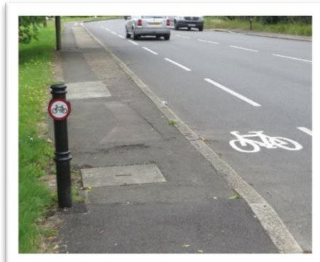
Gaston Bridge Road, cycle track to cycle lane The 'No Cycling' sign has been used to show the end of track, as the sign can be smaller.
