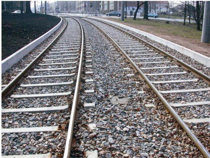
Chemnitz, Goethestraße before naturation
