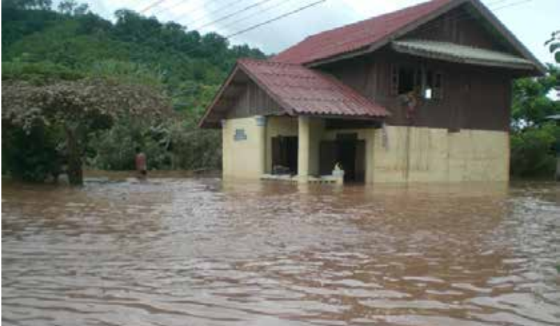
Inundated house (top) and part of Highway No. 13 (bottom) during the 8 August 2012 flooding
