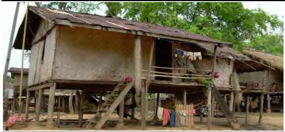
Figure 5.34 Houses at Ban Hat Gniun
