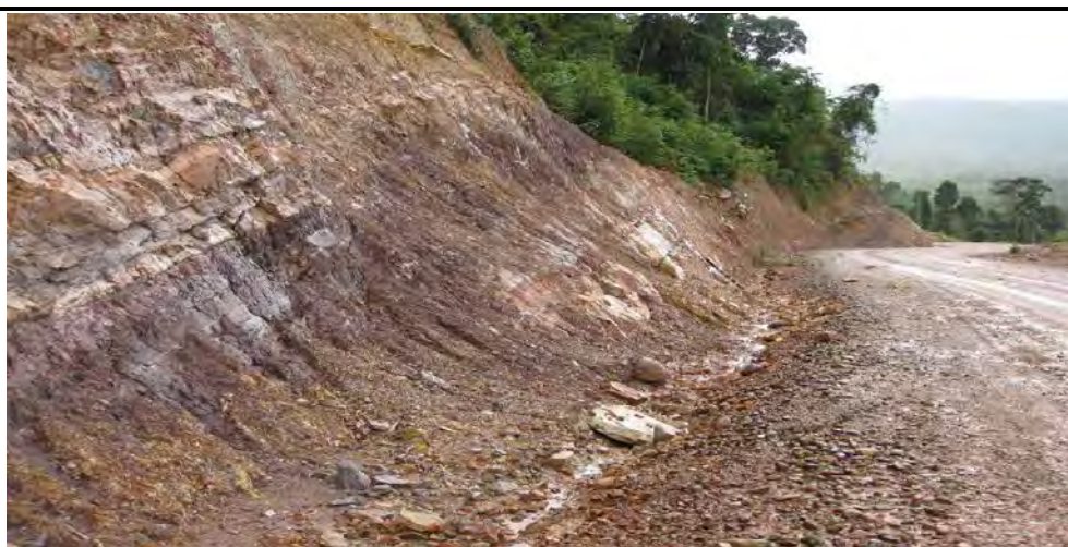
Figure 6.2 Water Drainage Channel Provided along an Elevated Unpaved Road
