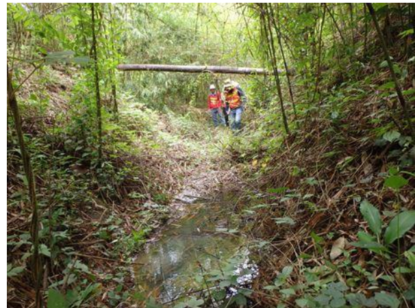
Plate 3-2: Houay Keehia (New Temporary Access Road)
