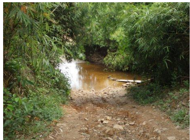
Plate 3-4: Houay Soup Noy (Existing Access Road Upgrade)
