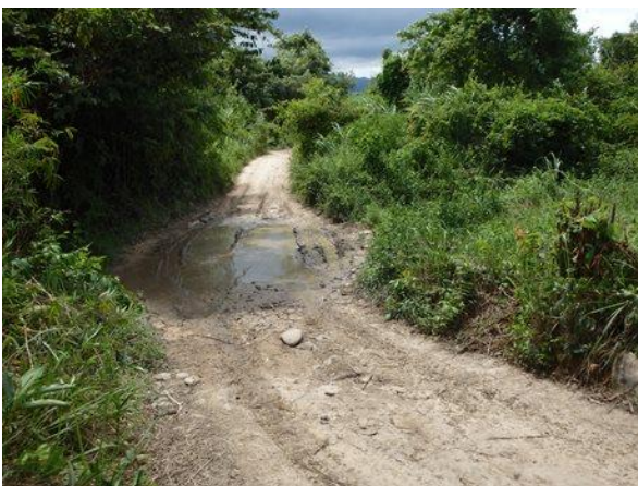
Plate 3-3: Houay Na (Existing Access Road Upgrade)
