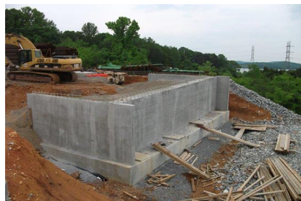
Plate 2-6: Example of the proposed Bridge Abutment
